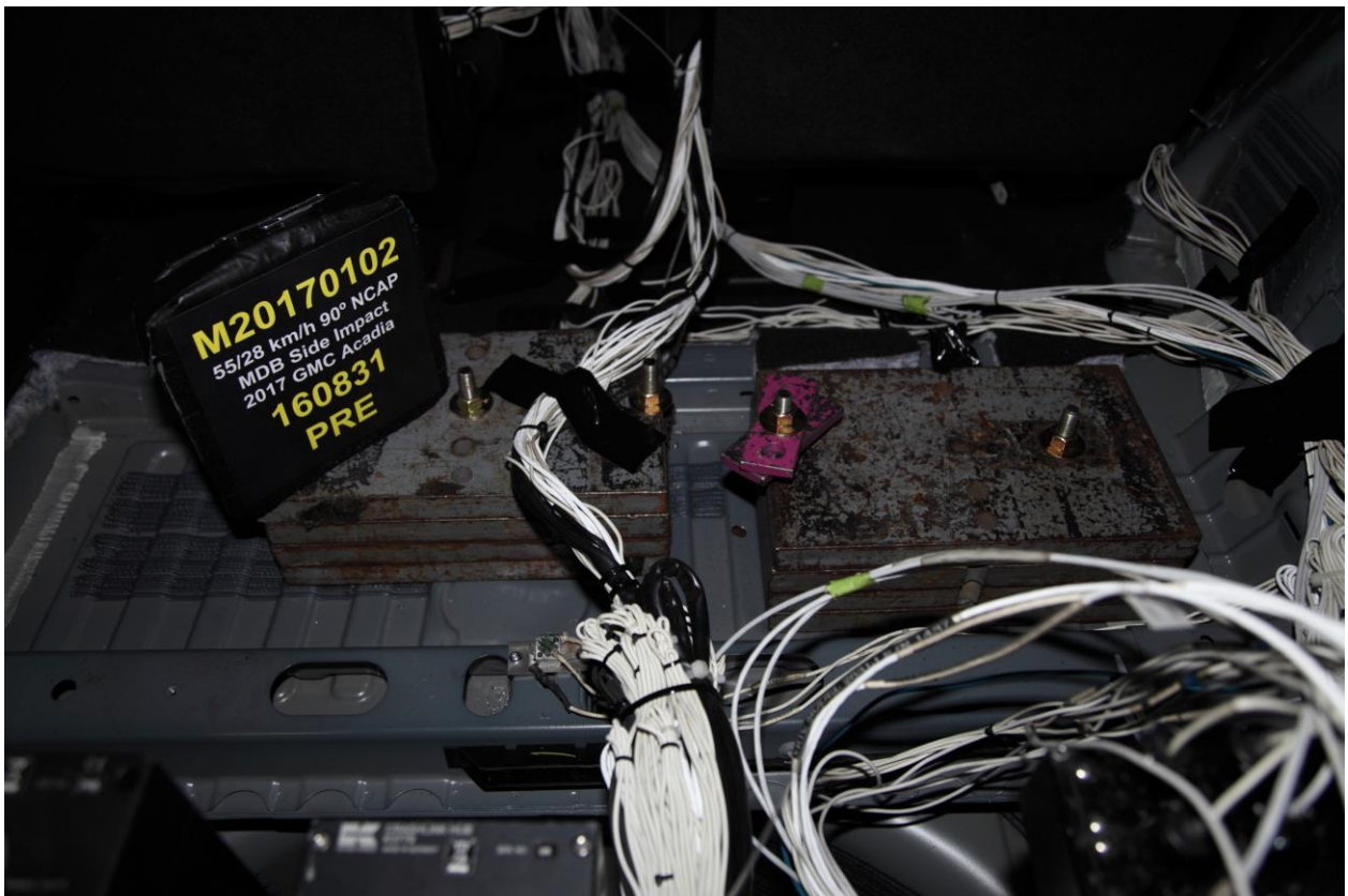
094c Pre-Test Ballast View 4
