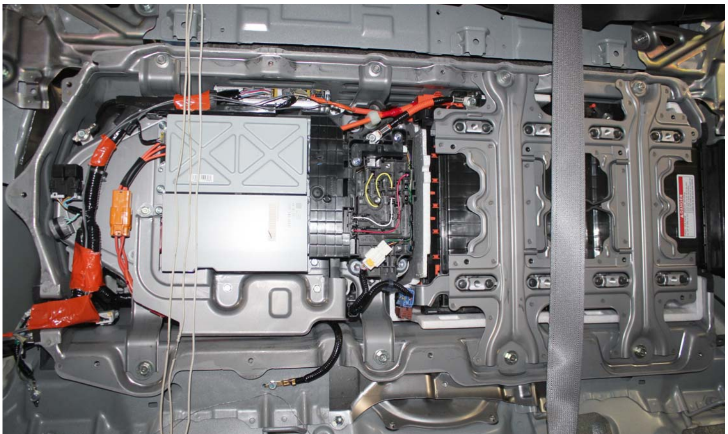
Pre-Impact View of Propulsion Battery
