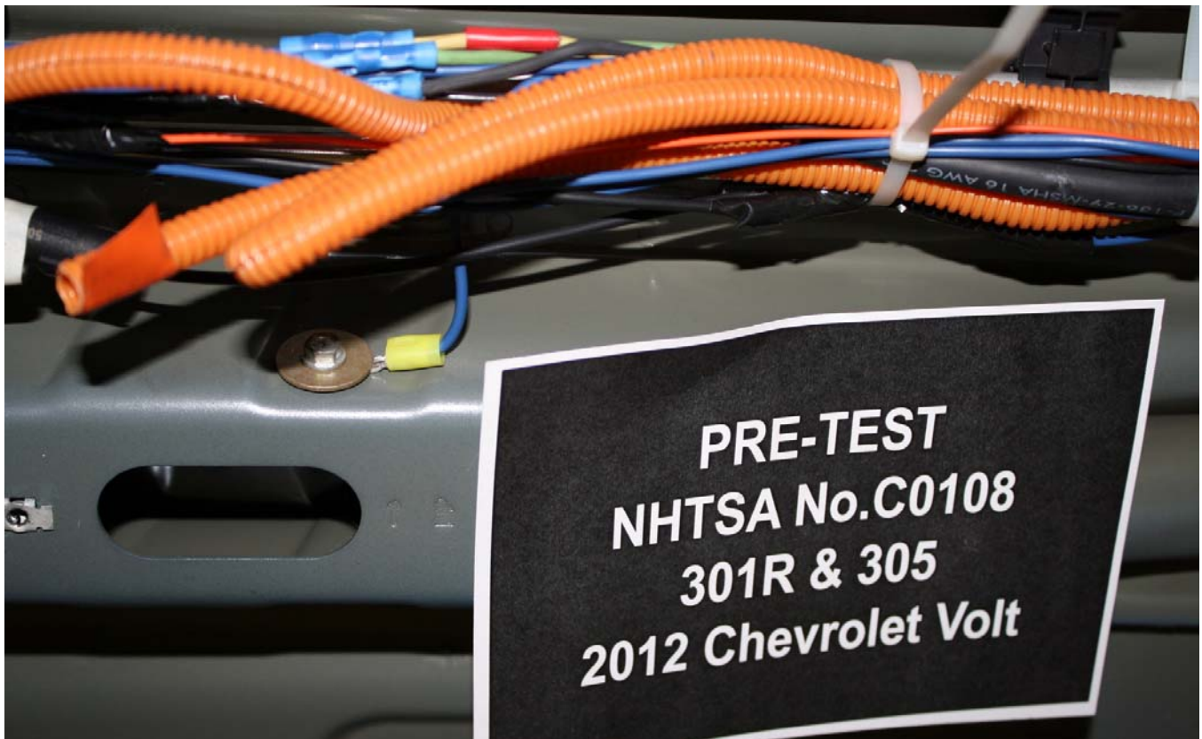
Figure A-61: Pre-Impact View of Ground Lead Attached
