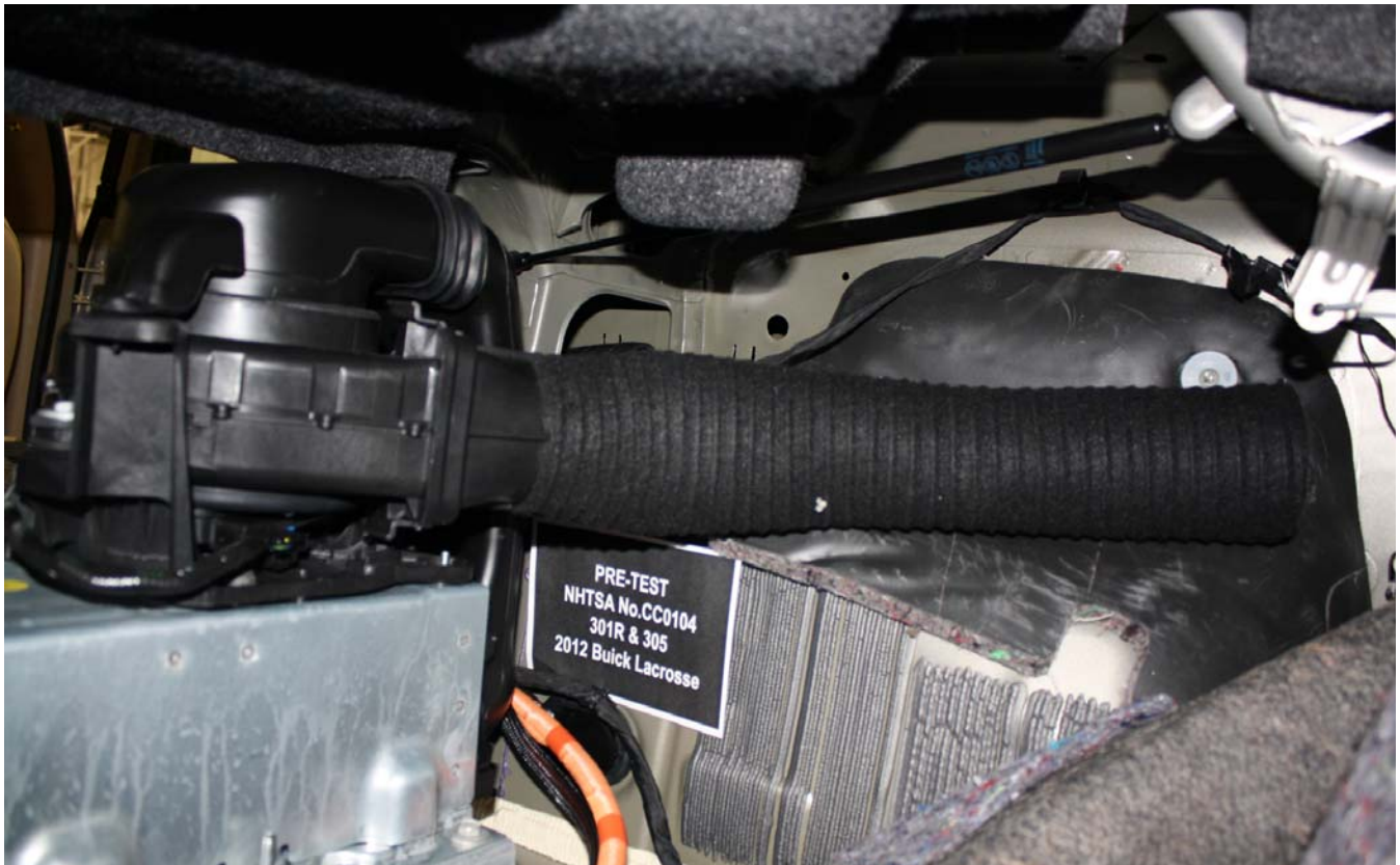
Figure A-59: Pre-Impact View Propulsion Battery Venting System(s)
