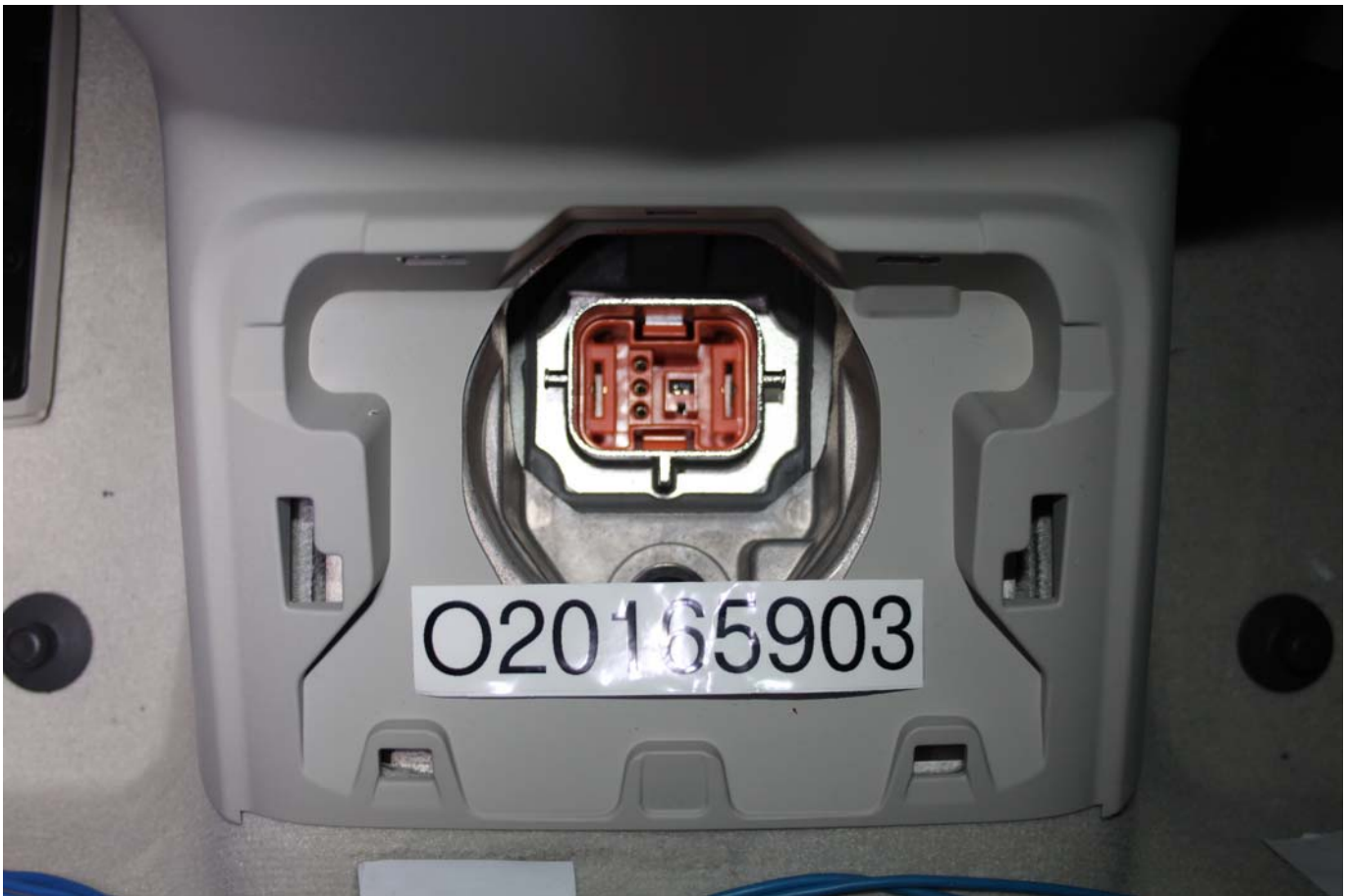
Photo No. 007 - Manual High Voltage Service Disconnect Removed
