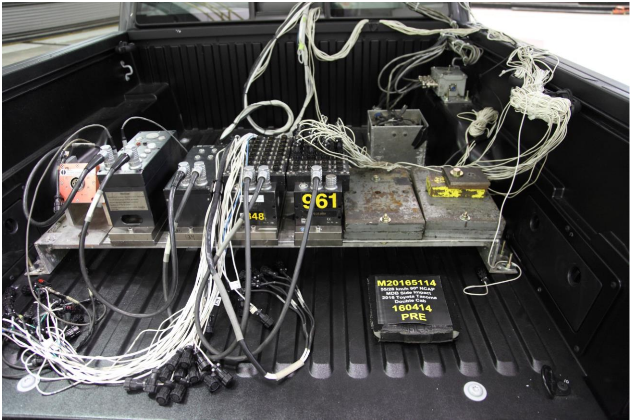
094 Pre-Test Ballast View
