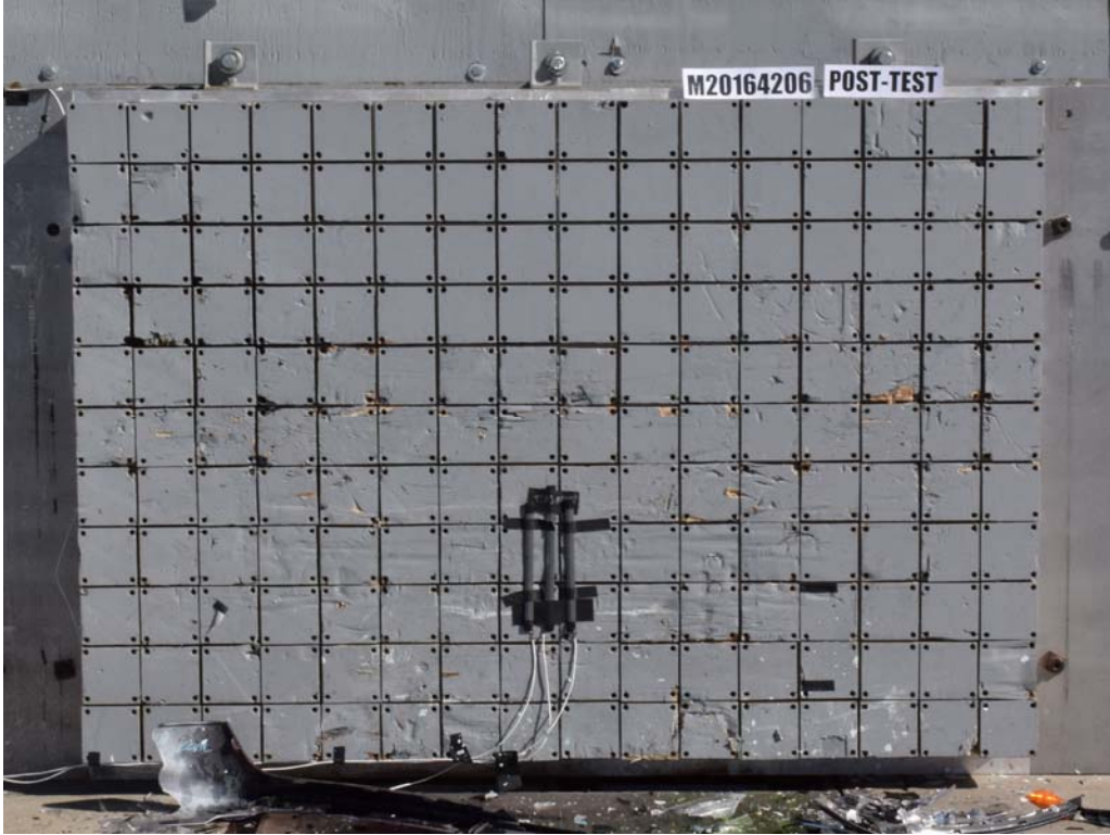
FIGURE 3. Post-Test Load Cell Wall
