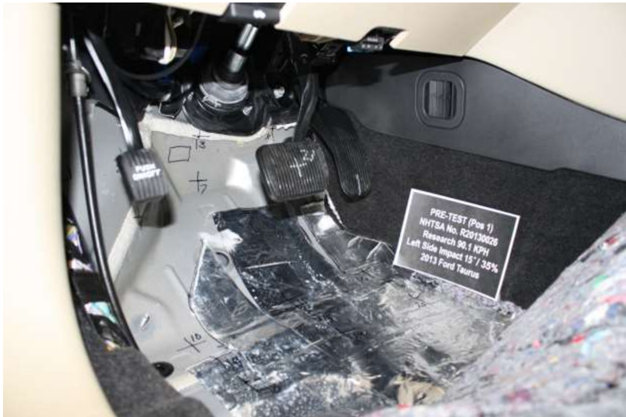
No. 048 Pre-Test View of Driver Floor pan at Left sill level, w/o carpet
