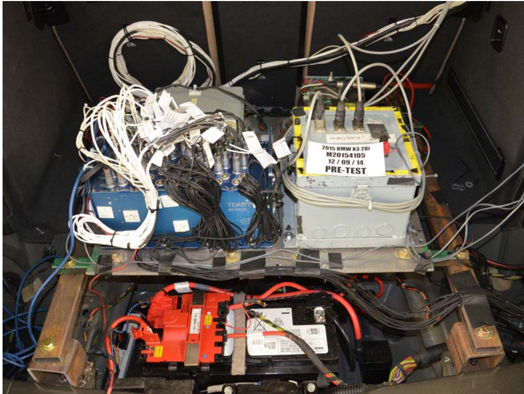
FIGURE 61. Pre-Test Ballast View
