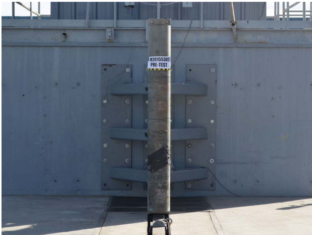
FIGURE 57. Pre-Test Pole Barrier Front View
