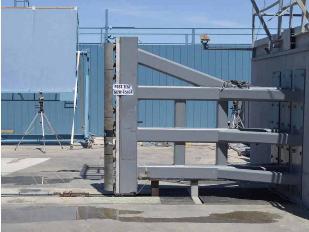
FIGURE 60. Post-Test Pole Barrier Side View
