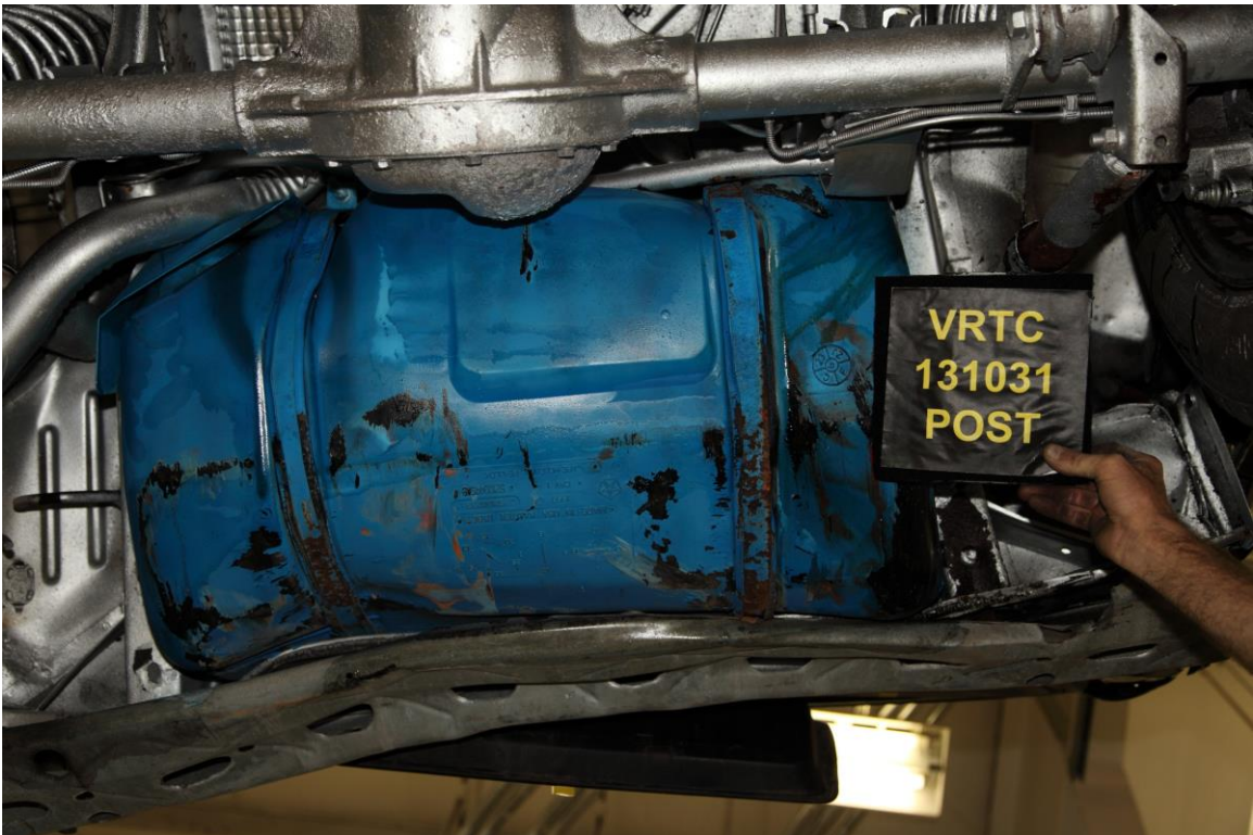
Figure A-20 Post-Test Target Vehicle Fuel Tank Close-up View
