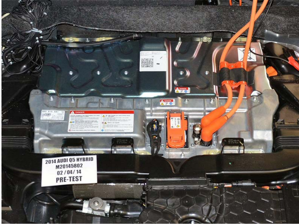
FIGURE 9a. Pre-Impact View of Propulsion Battery
