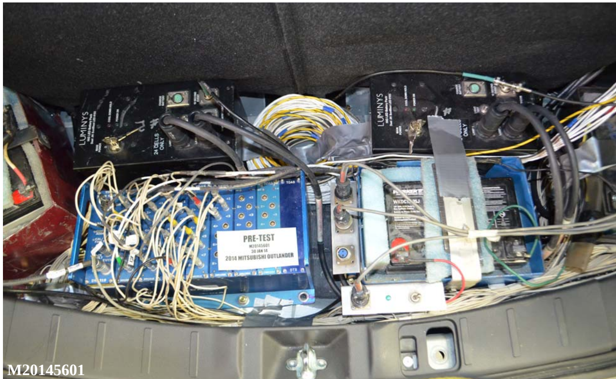
Figure 061: Pre-Test Ballast View
