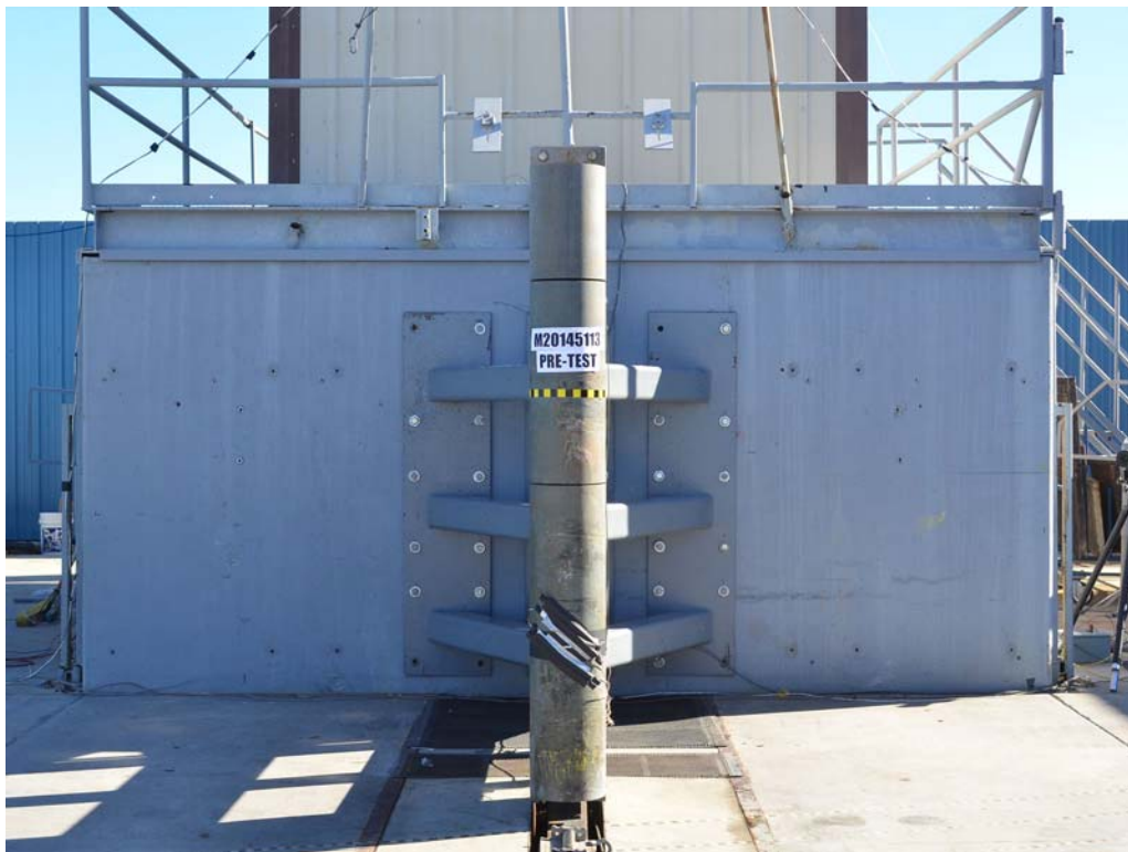
FIGURE 57. Pre-Test Pole Barrier Front View
