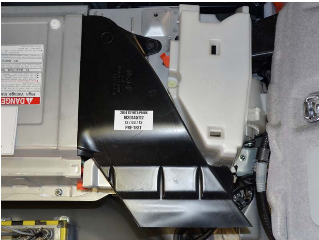
FIGURE 19a. Pre-Impact View of Propulsion Battery Venting System
