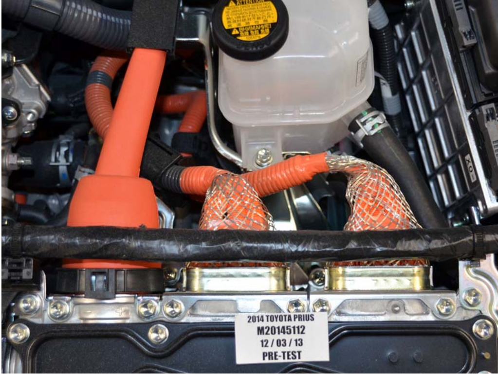
FIGURE 18. Pre-Impact View of High Voltage Interconnects
