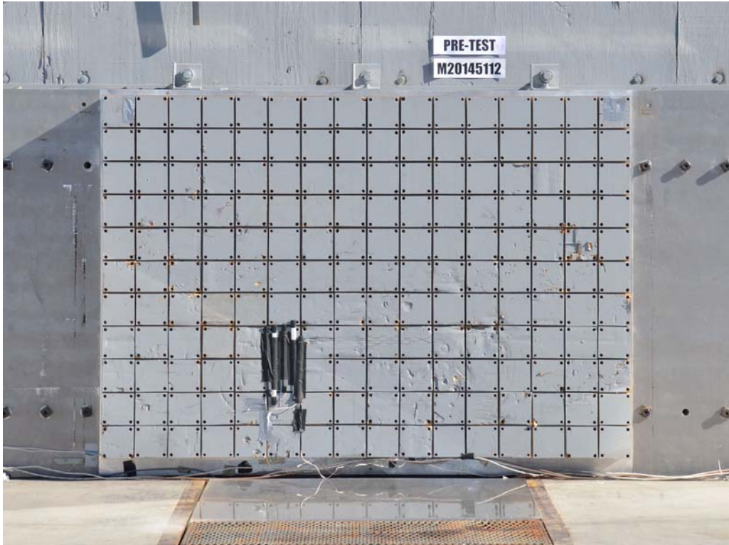
FIGURE 2. Load Cell Wall
