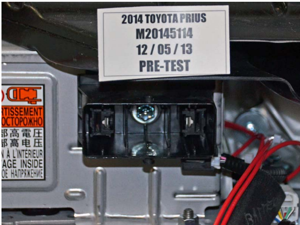
FIGURE 8. Manual High Voltage Service Disconnect Removed
