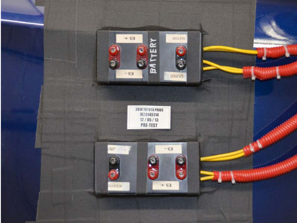
FIGURE 24. Pre-Impact View of Installed Test Interface Port
