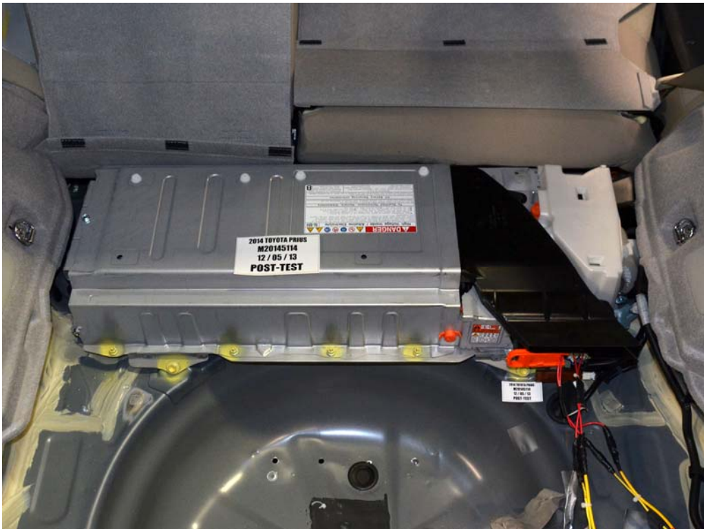
FIGURE 11. Post-Impact Rear View of Propulsion Battery
