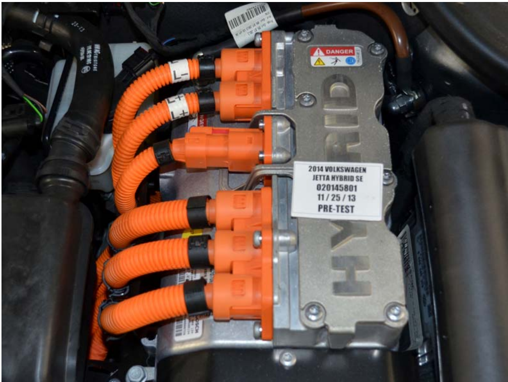
FIGURE 18. Pre-Impact View of High Voltage Interconnect(s)
