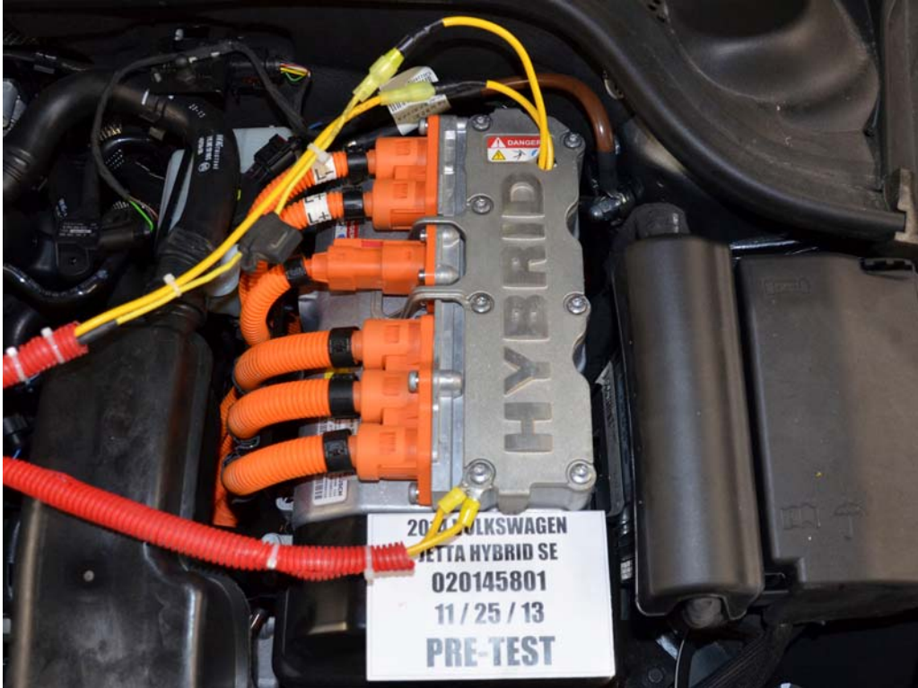
FIGURE 22. Pre-Impact View of High Voltage Leads Attached
