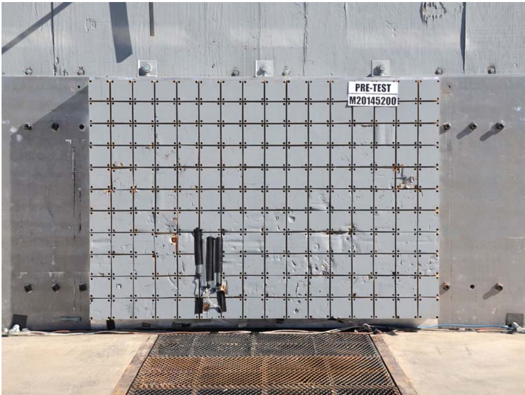
FIGURE 2. Load Cell Wall
