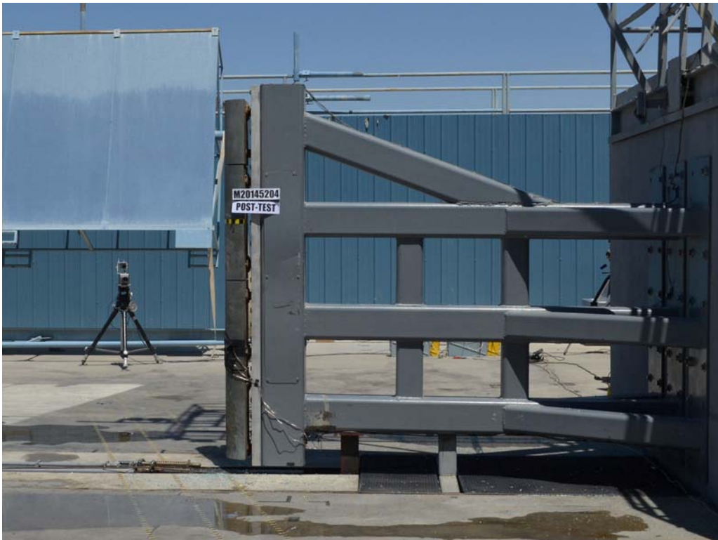
FIGURE 60. Post-Test Pole Barrier Side View
