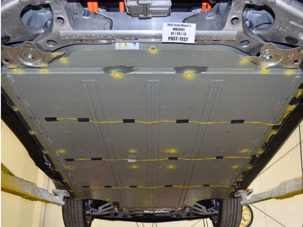
FIGURE 11. Post-Impact Rear View of Propulsion Battery
