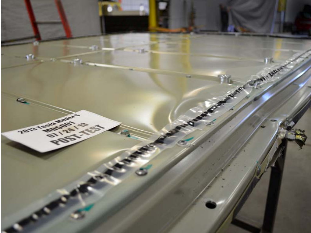
FIGURE 36b. Post-Impact View of Propulsion Battery Component Intrusion
