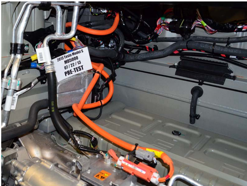
FIGURE 18. Pre-Impact View of High Voltage Interconnect(s)
