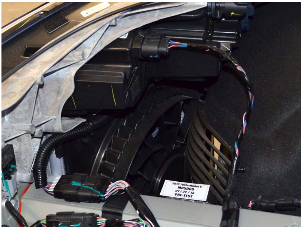
FIGURE 19. Pre-Impact View of Battery Venting System(s)
