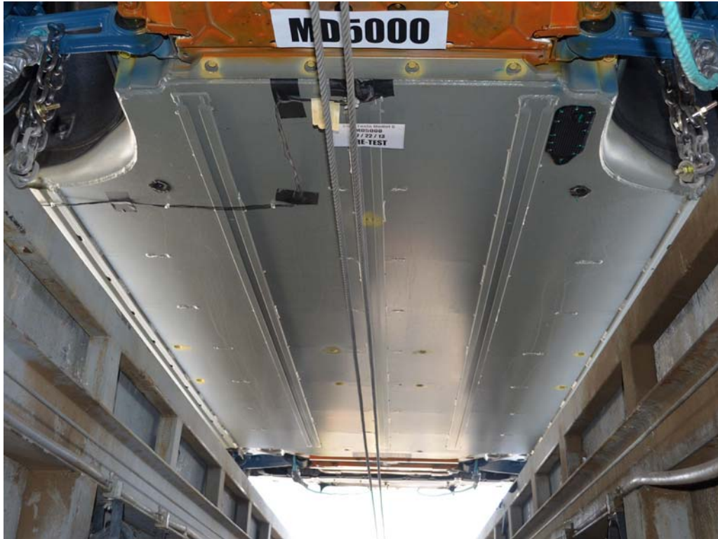
FIGURE 9a. Pre-Impact View of Propulsion Battery
