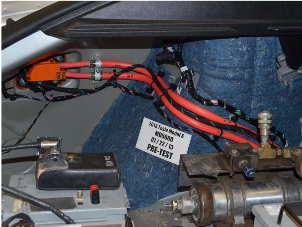
FIGURE 18g. Pre-Impact View of High Voltage Interconnect(s)
