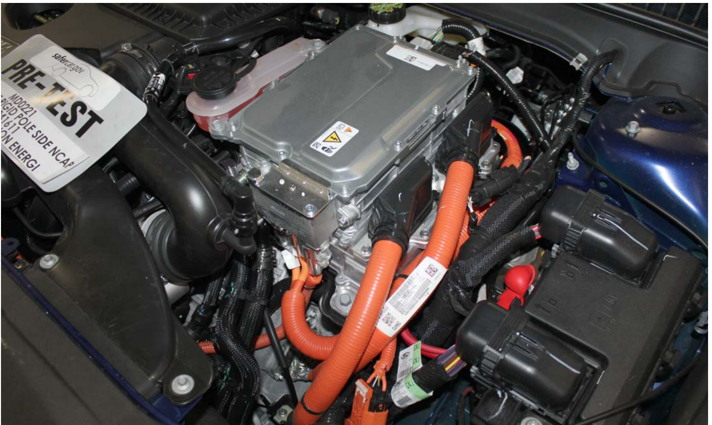
No. 002 Power Inverter Warning Label
