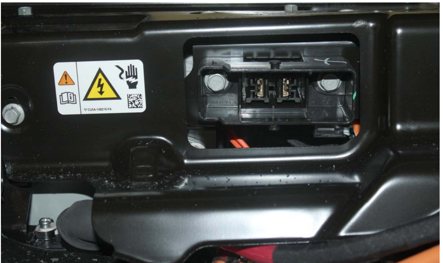
No. 007 Manual High Voltage Service Disconnect Removed
