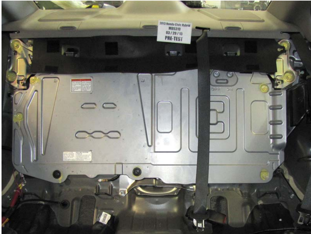
FIGURE 9. Pre-Impact View of Propulsion Battery
