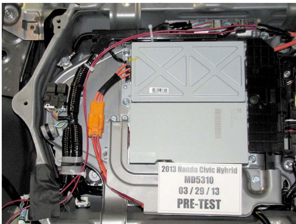
FIGURE 22. Pre-Impact View of High Voltage Leads Attached
