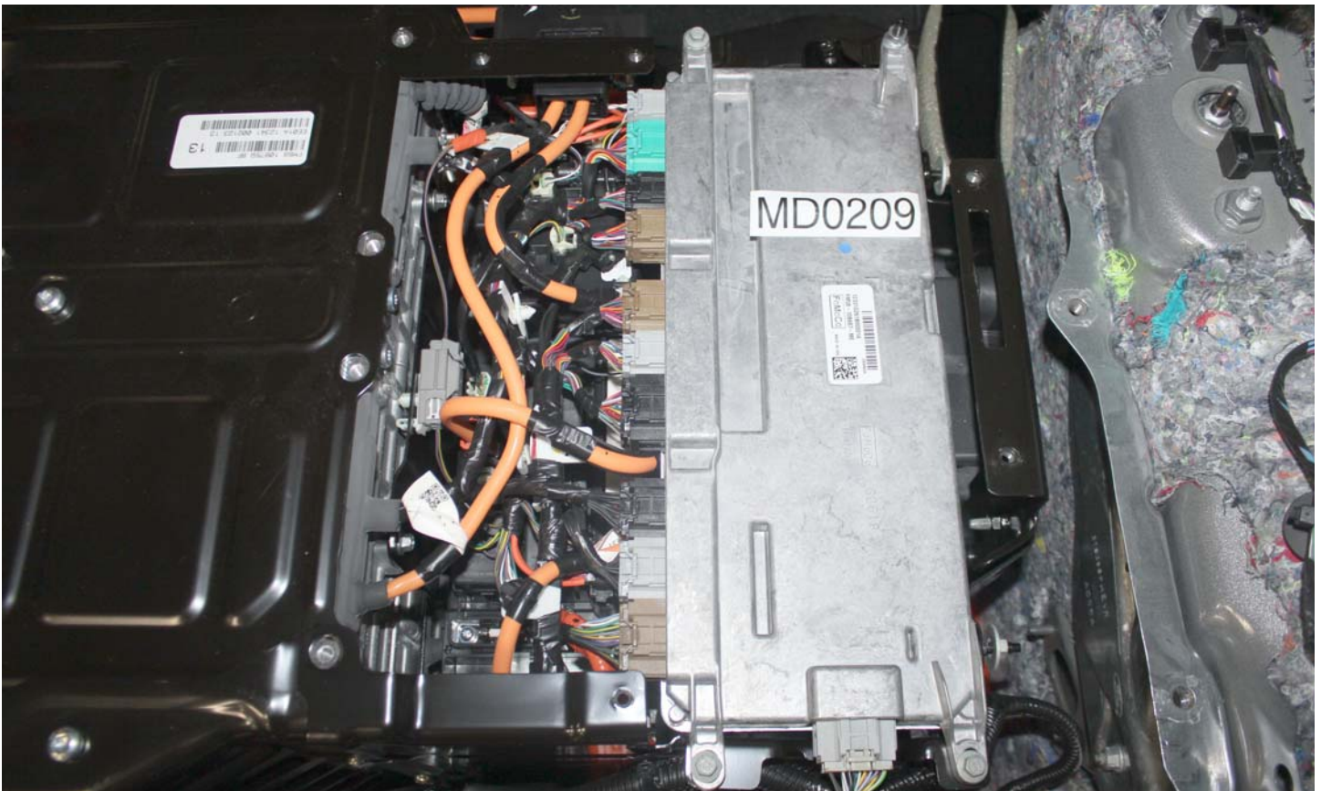
No. 018 Pre-Impact View of High Voltage Interconnect(s)
