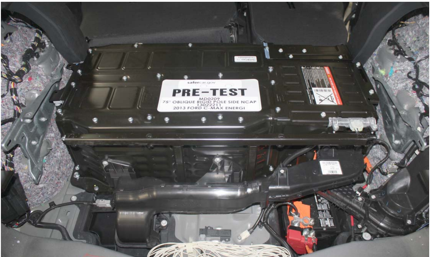
No. 009 Pre-Impact View of Propulsion Battery
