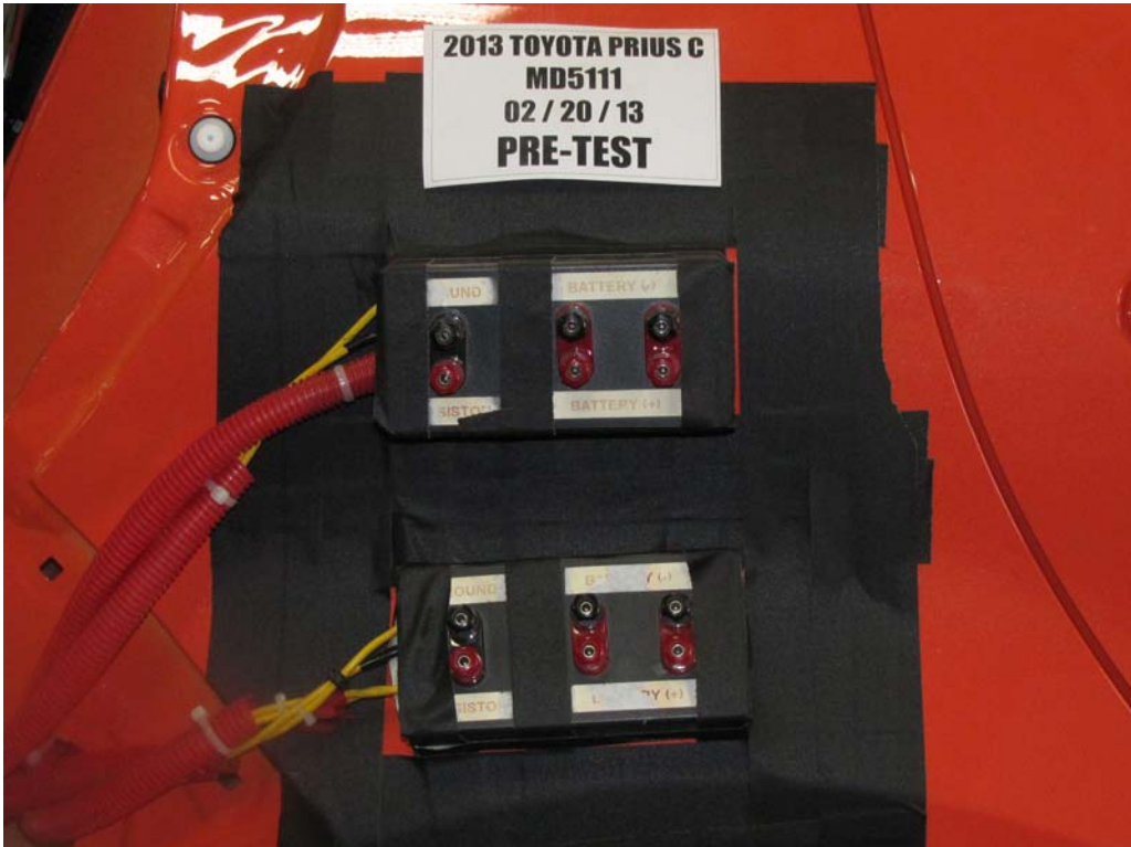
FIGURE 24. Pre-Impact View of Installed Test Interface Port
