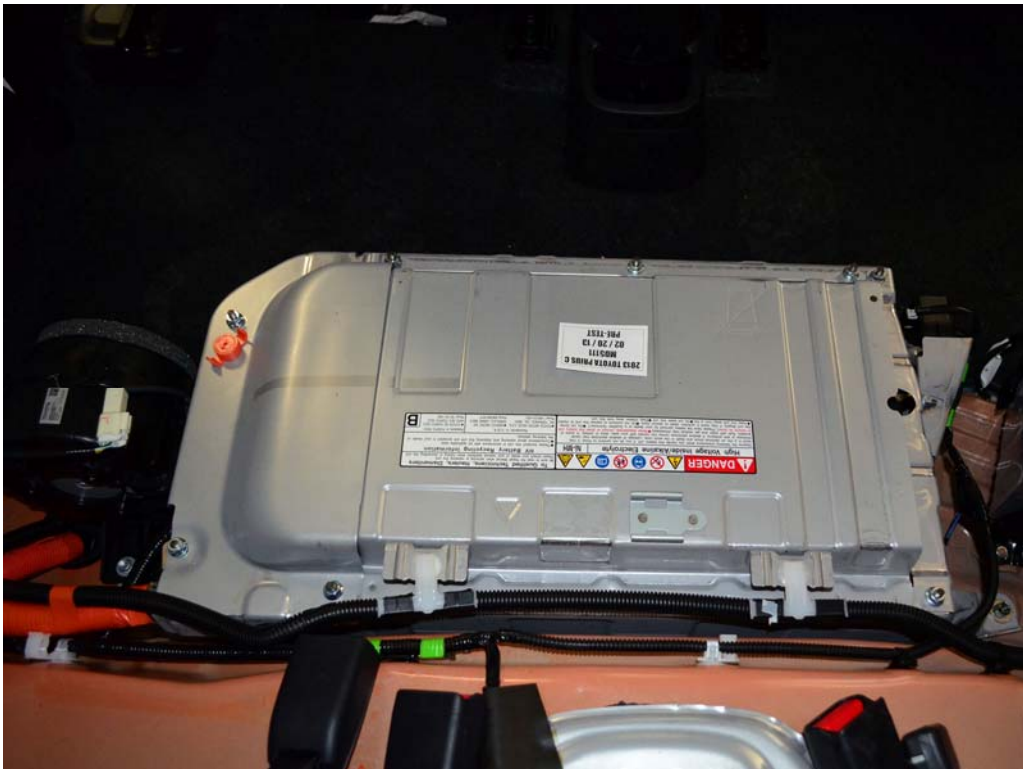
FIGURE 9a. Pre-Impact View of Propulsion Battery
