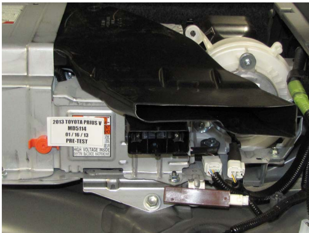
FIGURE 8. Manual High Voltage Service Disconnect Removed
