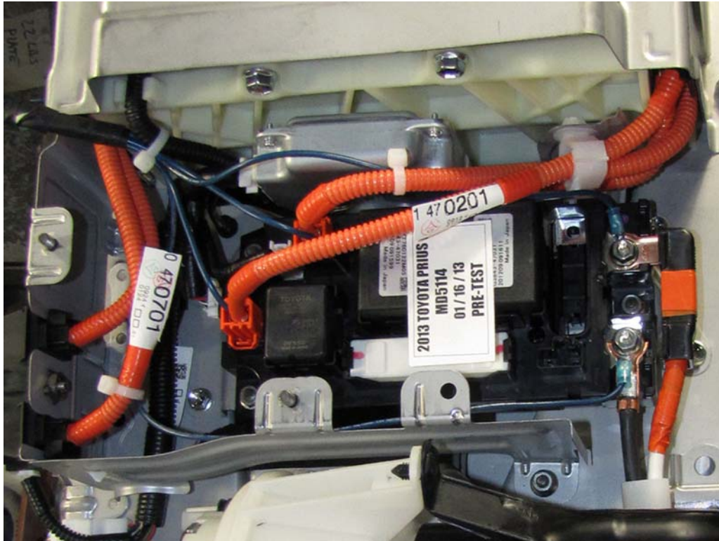
FIGURE 22. Pre-Impact View of High Voltage Leads Attached
