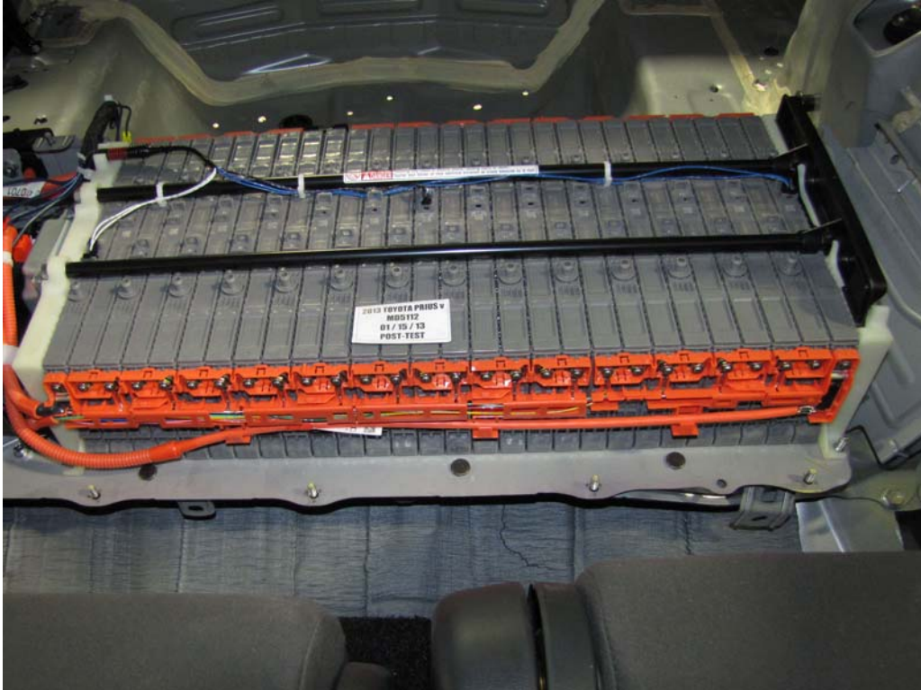
FIGURE 15. Post-Impact View of Propulsion Battery Modules
