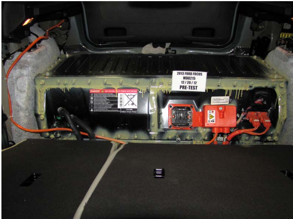
FIGURE 9. Pre-Impact View of Propulsion Battery
