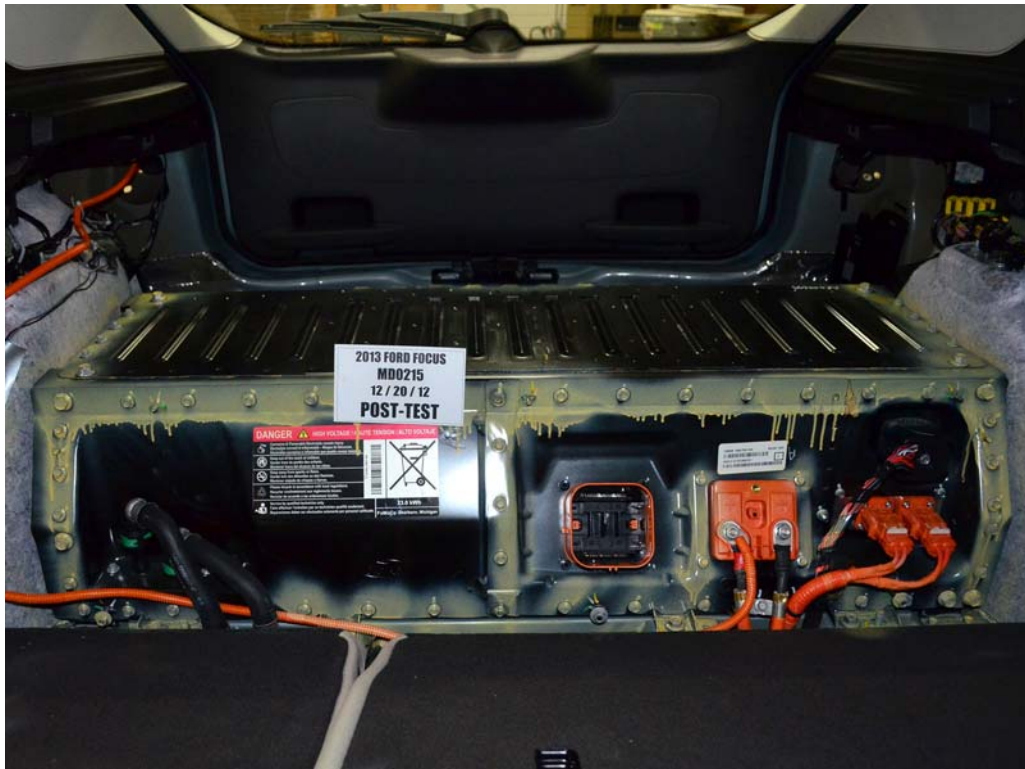
FIGURE 10. Post-Impact Front View of Propulsion Battery
