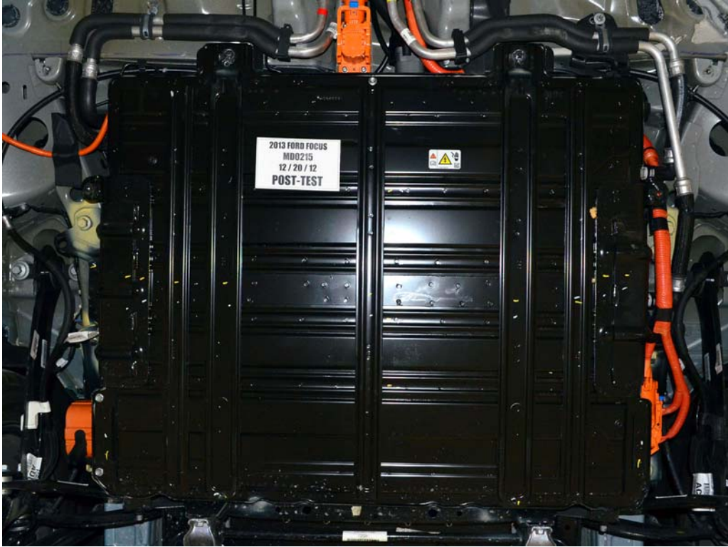
FIGURE 10a. Post-Impact Front View of Propulsion Battery
