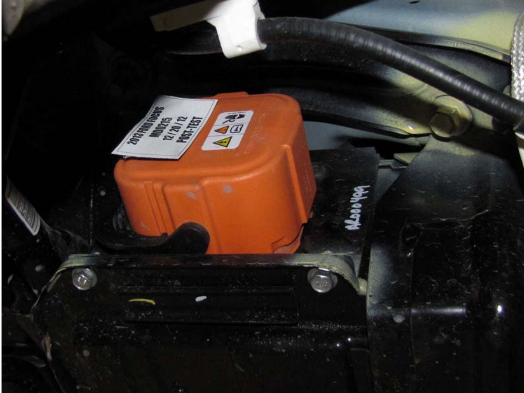
FIGURE 6a. Manual High Voltage Service Disconnect In Place
