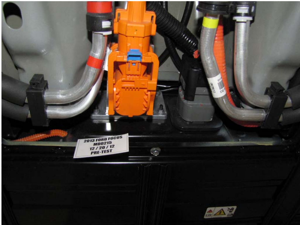
FIGURE 18b. Pre-Impact View of High Voltage Interconnect(s)
