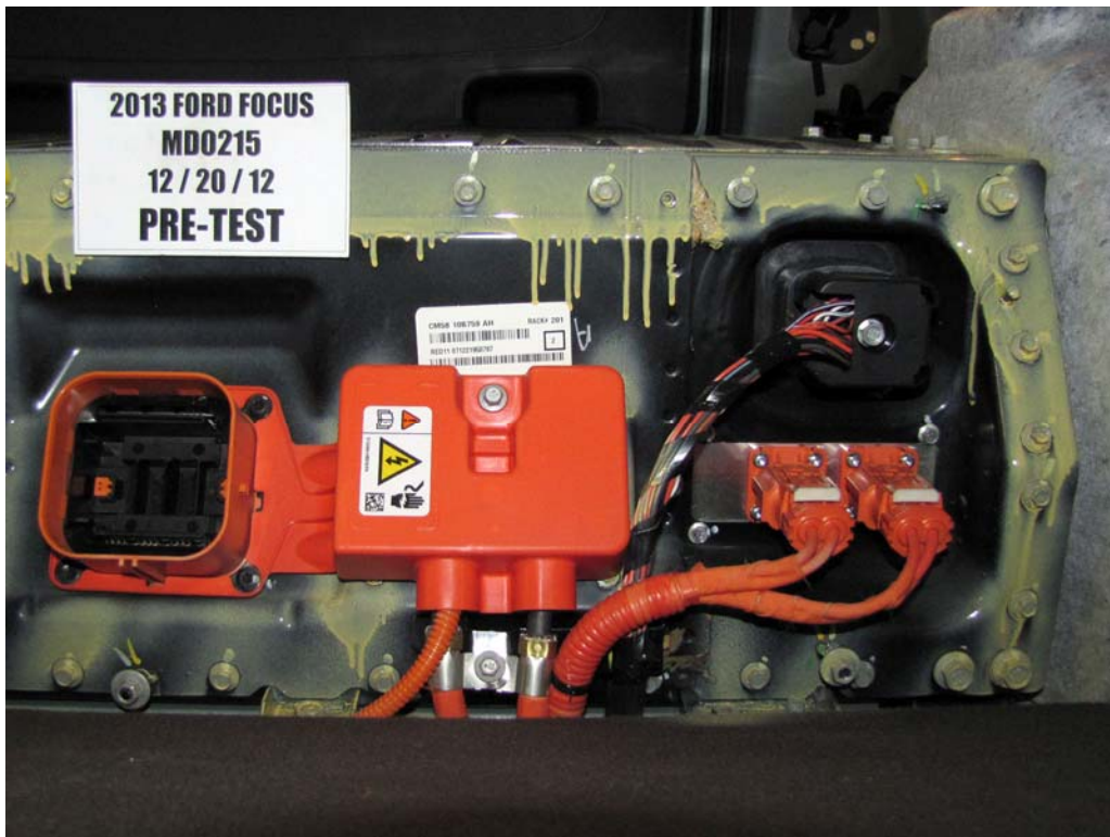
FIGURE 22. Pre-Impact View of High Voltage Leads Attached
