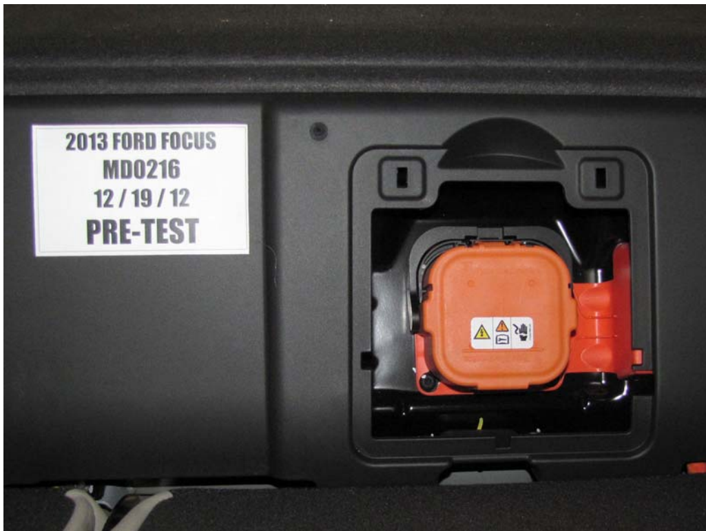
FIGURE 6. Manual High Voltage Disconnect In Place
