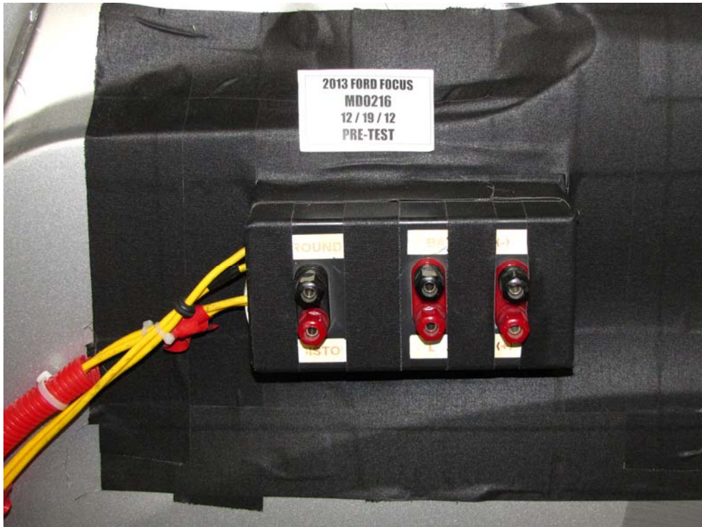
FIGURE 24. Pre-Impact View of Installed Test Interface Port
