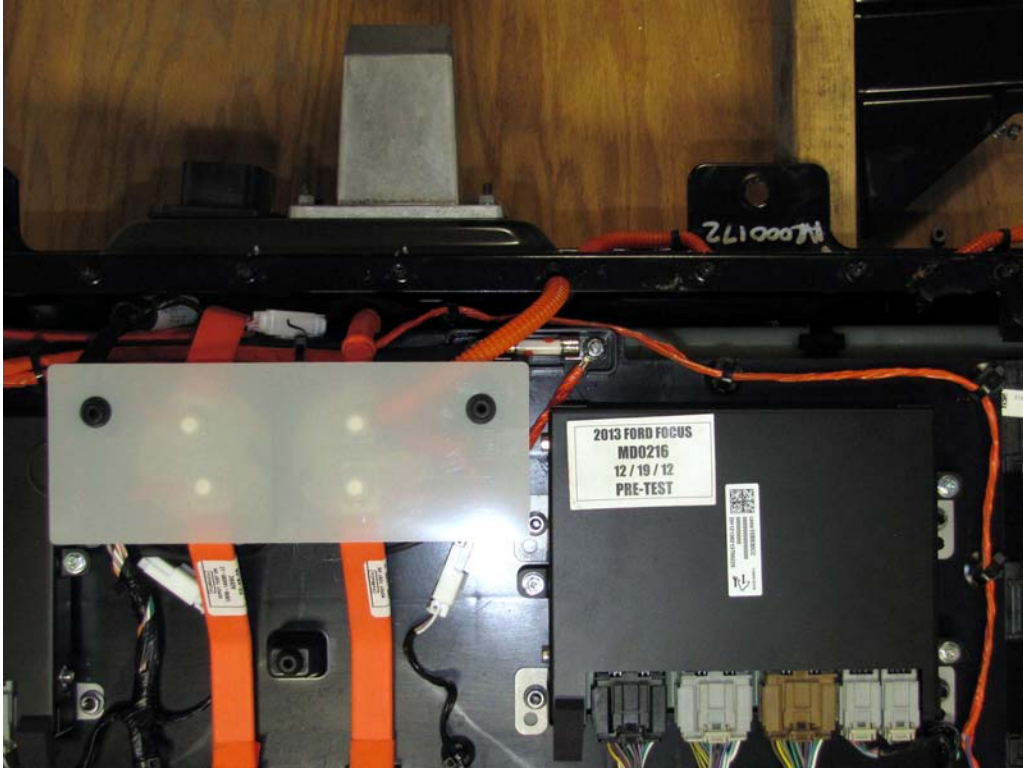
FIGURE 22a. Pre-Impact View of High Voltage Leads Attached
