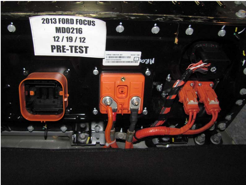
FIGURE 22. Pre-Impact View of High Voltage Leads Attached
