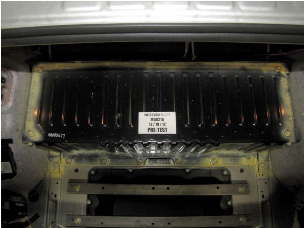
FIGURE 12. Pre-Impact View of Battery Box or Container Which hold Individual Battery Modules
