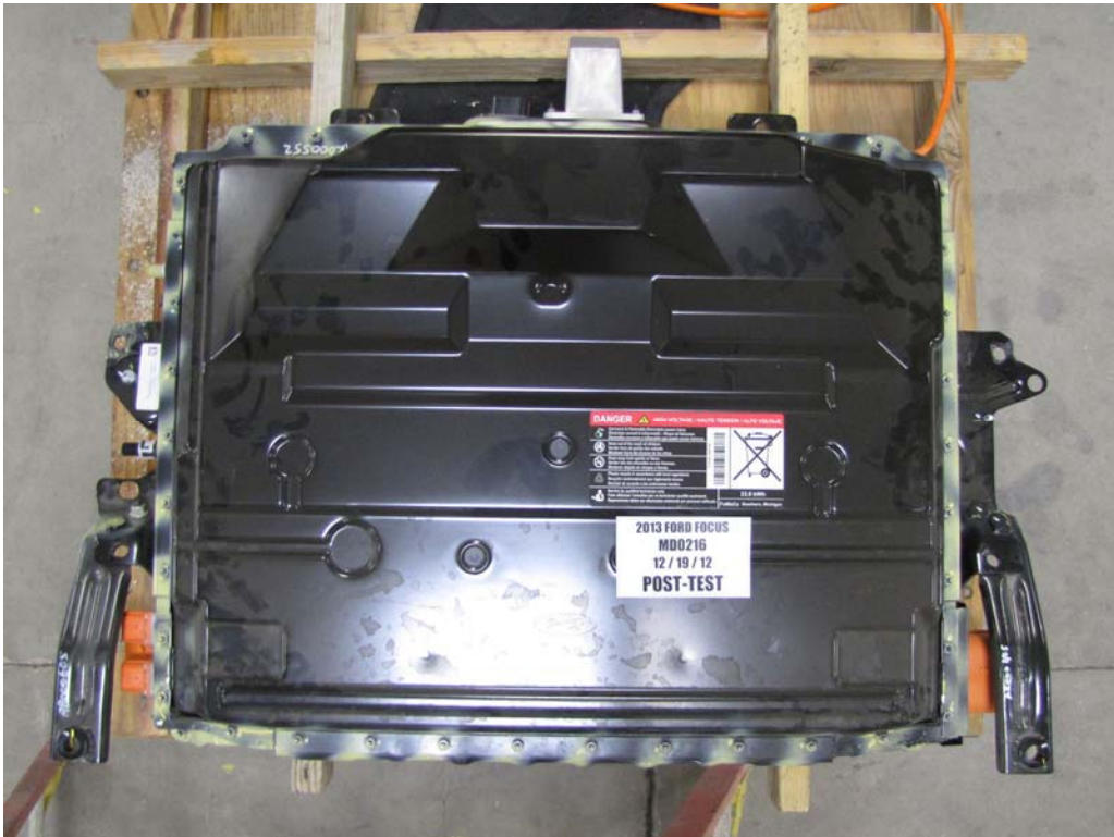
FIGURE 13a. Post-Impact View of Battery Box or Container Which hold Individual Battery Modules
