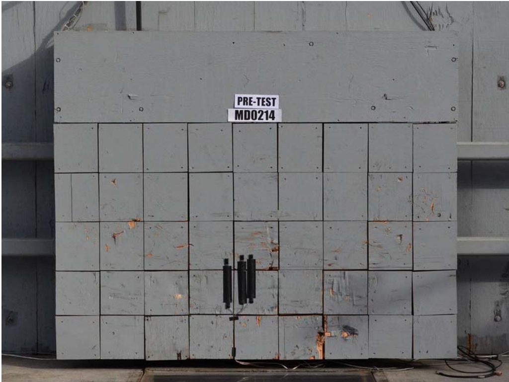
FIGURE 2. Load Cell Wall
