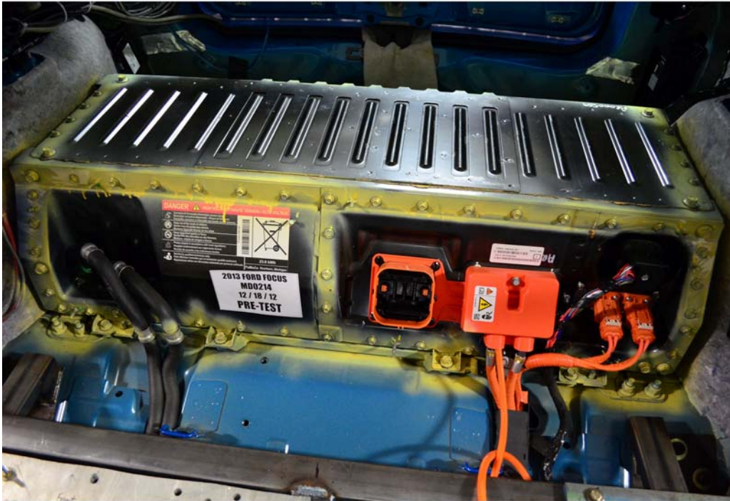
FIGURE 33. Pre-Impact View of Vehicle Passenger Compartment Adjacent to Propulsion Battery
