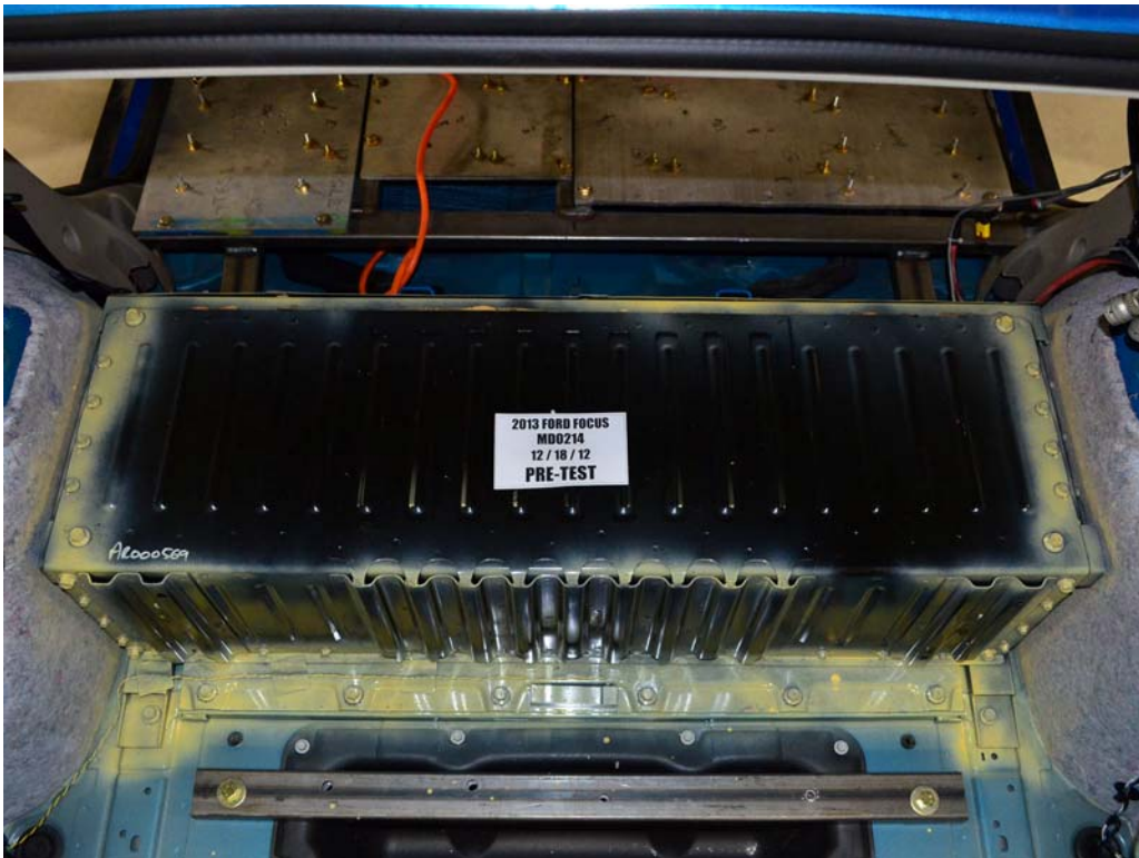
FIGURE 12. Pre-Impact View of Battery Box or Container Which hold Individual Battery Modules
