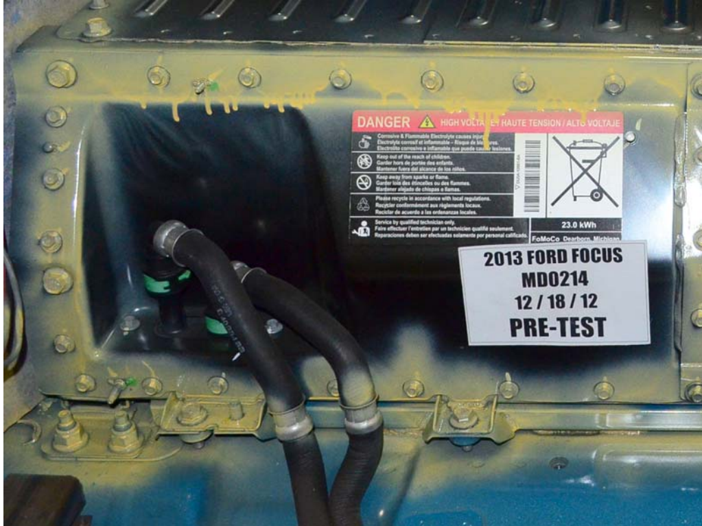
FIGURE 19a. Pre-Impact View of Propulsion Battery Venting System(s)
