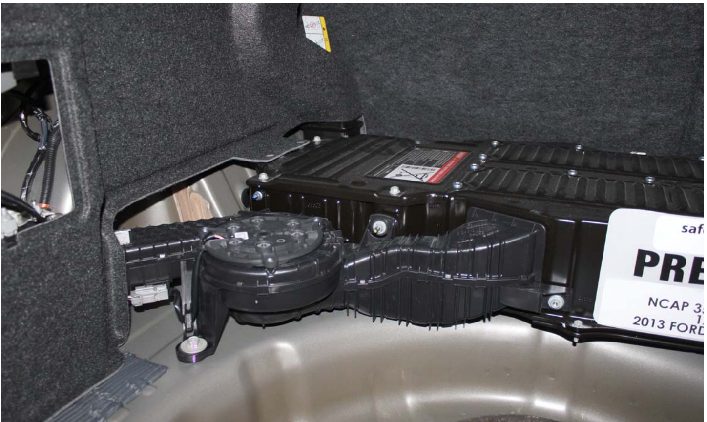
No. 019 Pre-Impact View Propulsion Battery Venting System(s)
