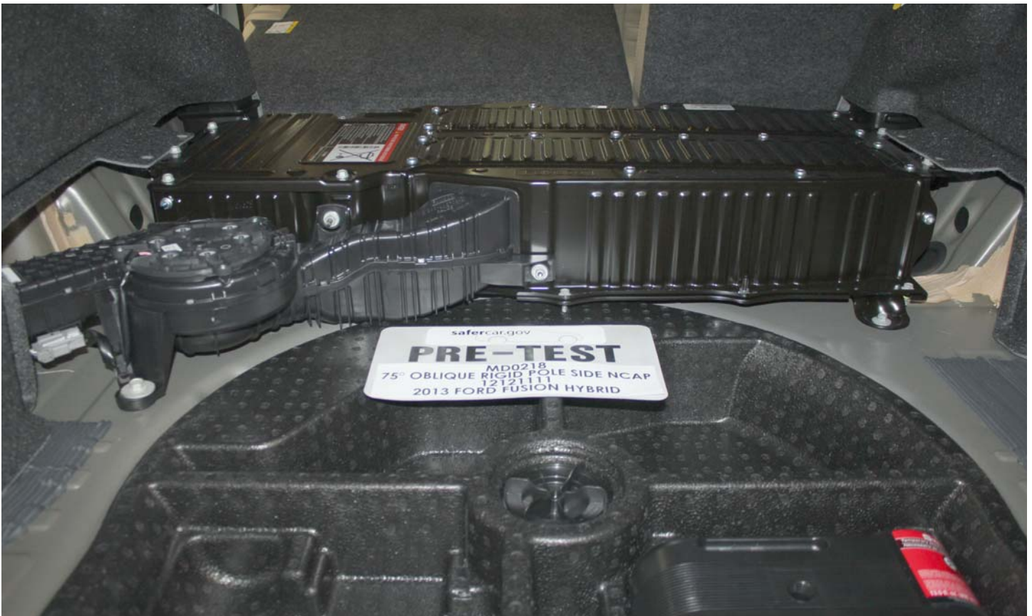
No. 012 Pre-Impact View of Battery Box(s) or Container(s) Which Holds Individual Battery Modules
