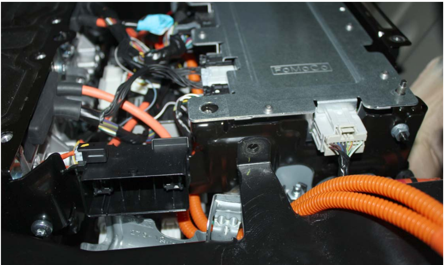
No. 007 Manual High Voltage Service Disconnect Removed
