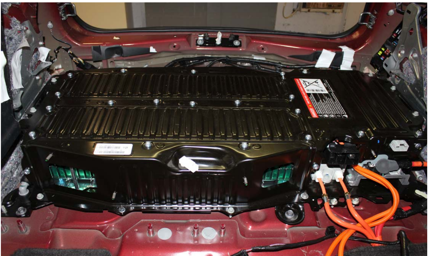
No. 010 Post-Impact Front View of Propulsion Battery
