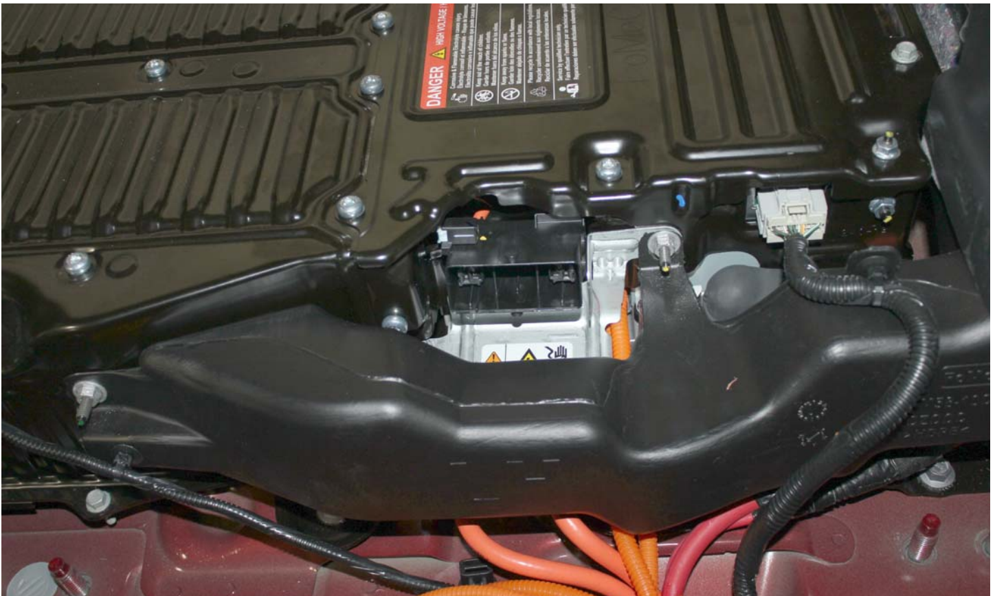
No. 007 Manual High Voltage Service Disconnect Removed
