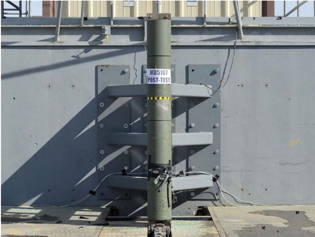
FIGURE 58. Post-Test Pole Barrier Front View
