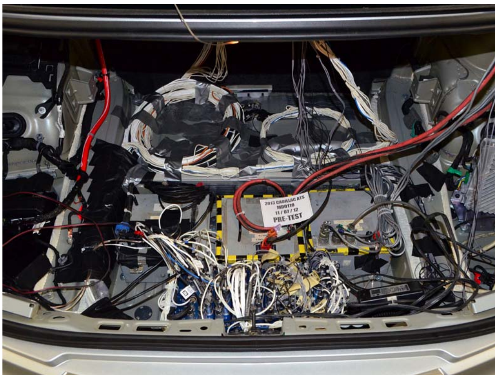
FIGURE 94. Pre-Test Ballast View
