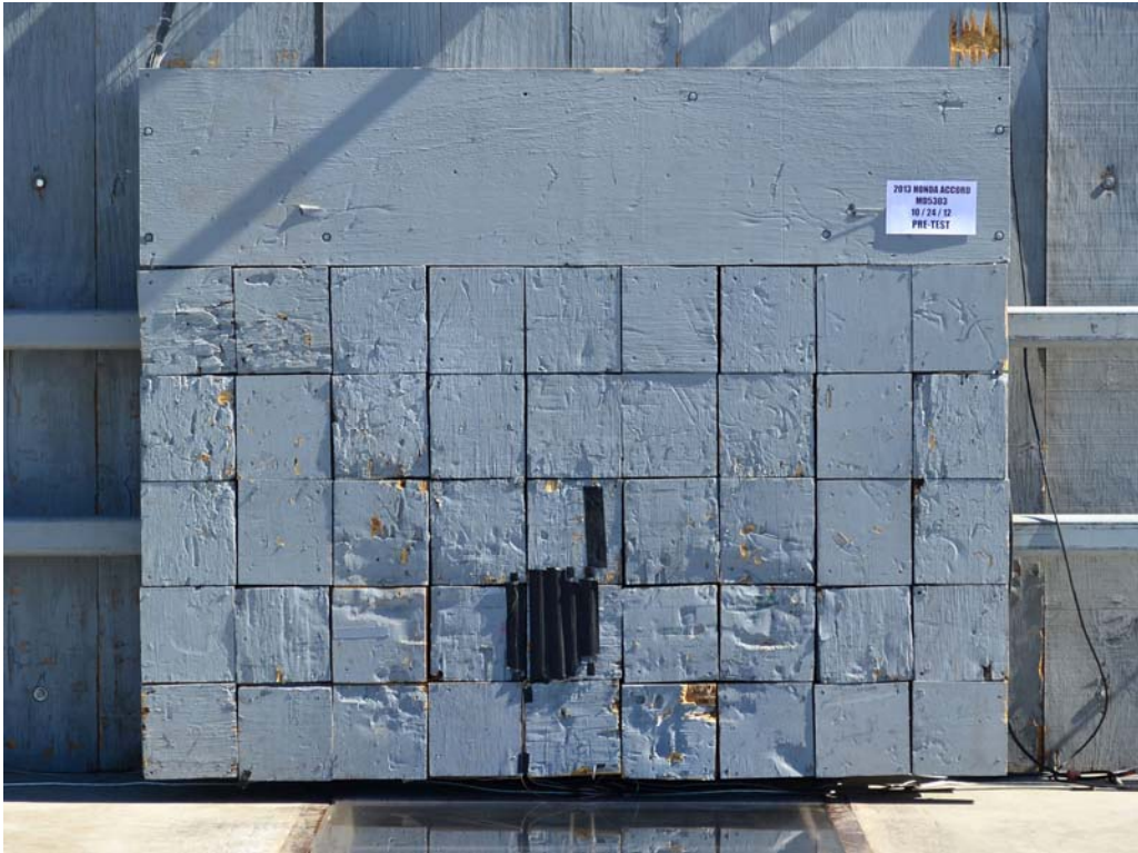
FIGURE 2. Load Cell Wall
