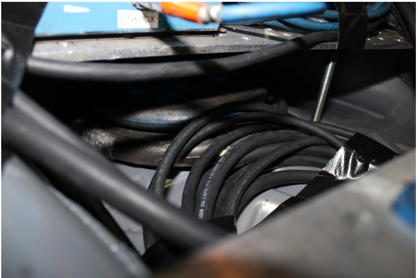
Pre-Test Ballast View
