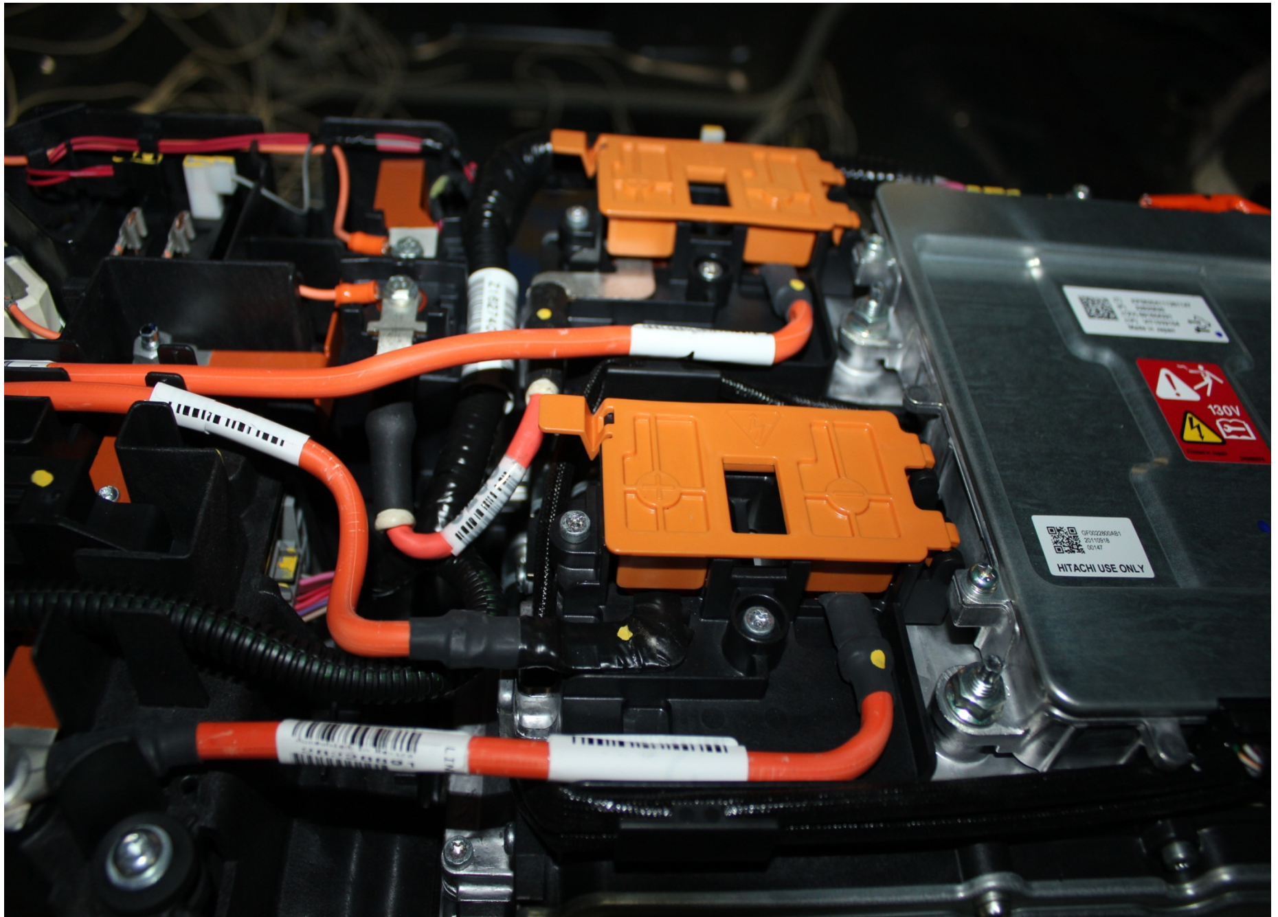
Pre-Test Positive and Negative Attachment Point to the Propulsion Battery System
