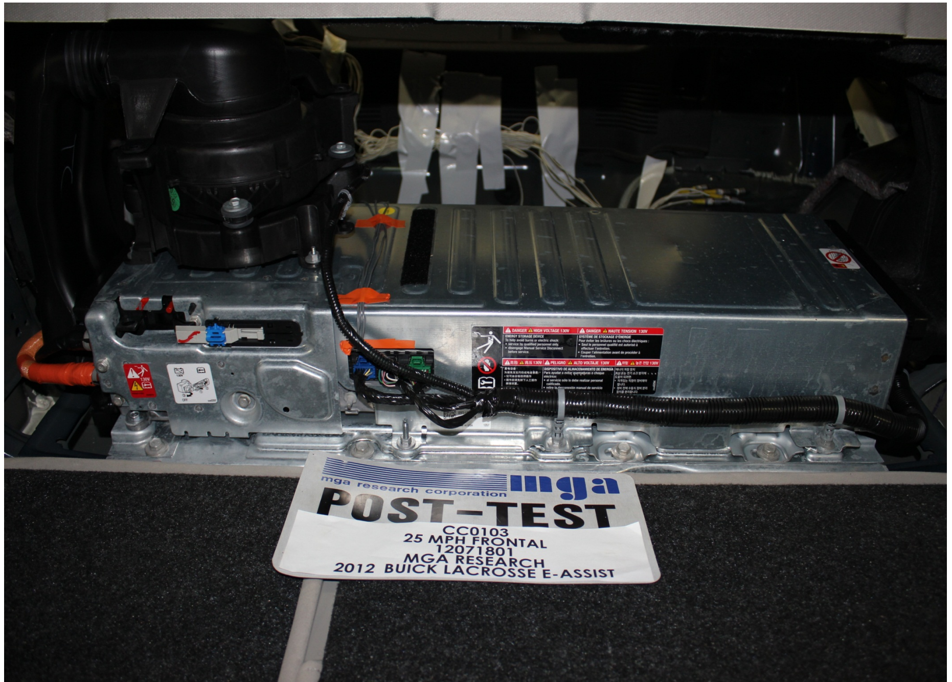
Post-Test Front View of Electrical Propulsion Battery
