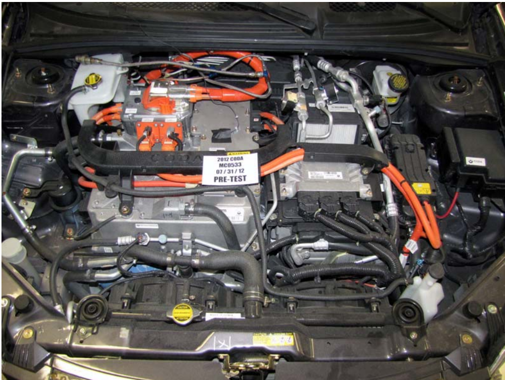
FIGURE 16. Pre-Impact View of Electric Propulsion Drive
