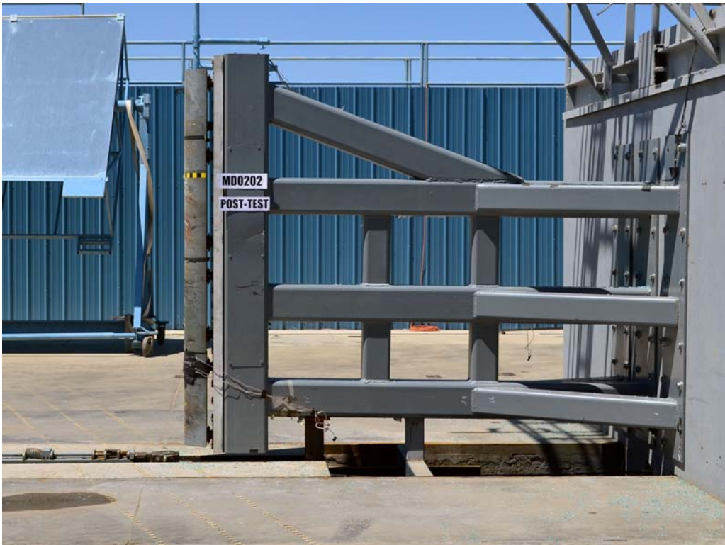
FIGURE 60. Post-Test Pole Barrier Side View
