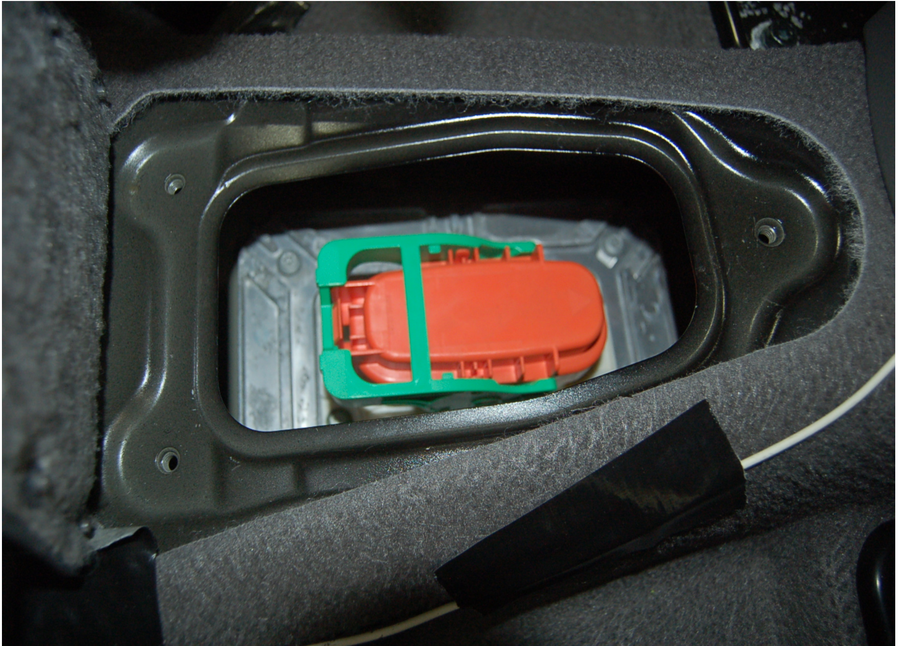
Manual High Voltage Service Disconnect Compartment View
