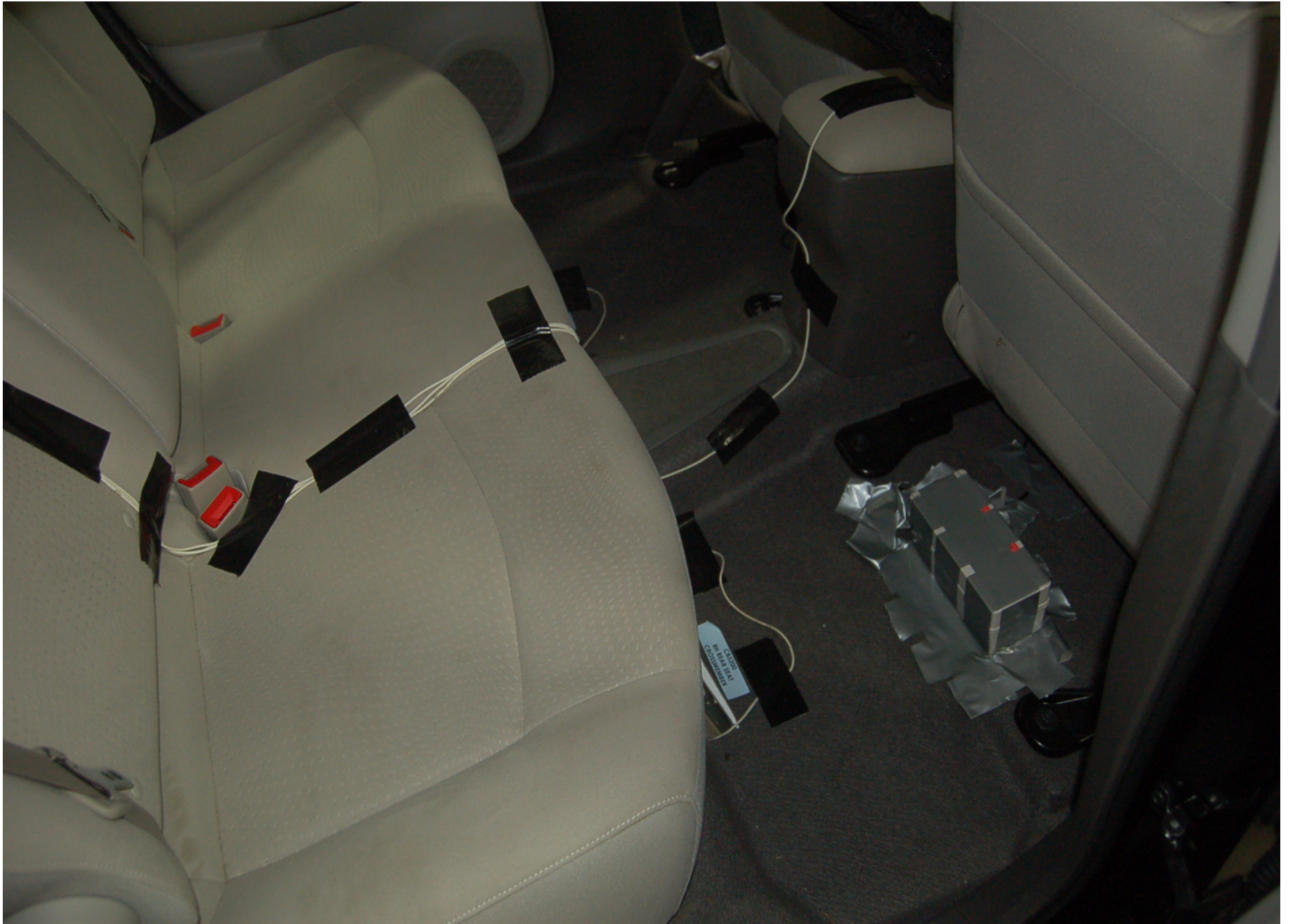
Manual High Voltage Service Disconnect
