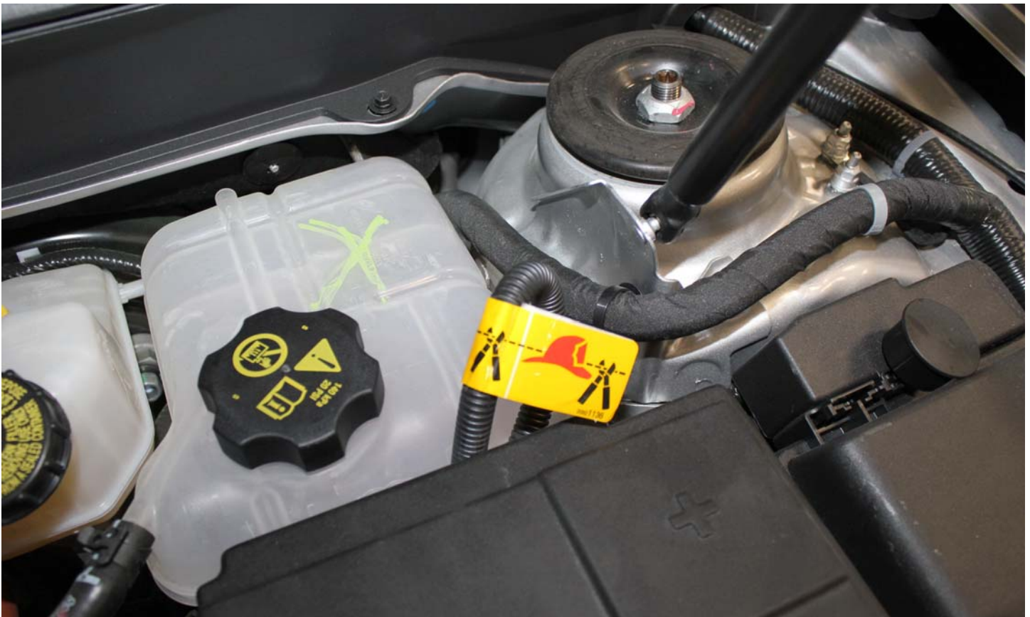
No. 004a First Responder Warning Location
