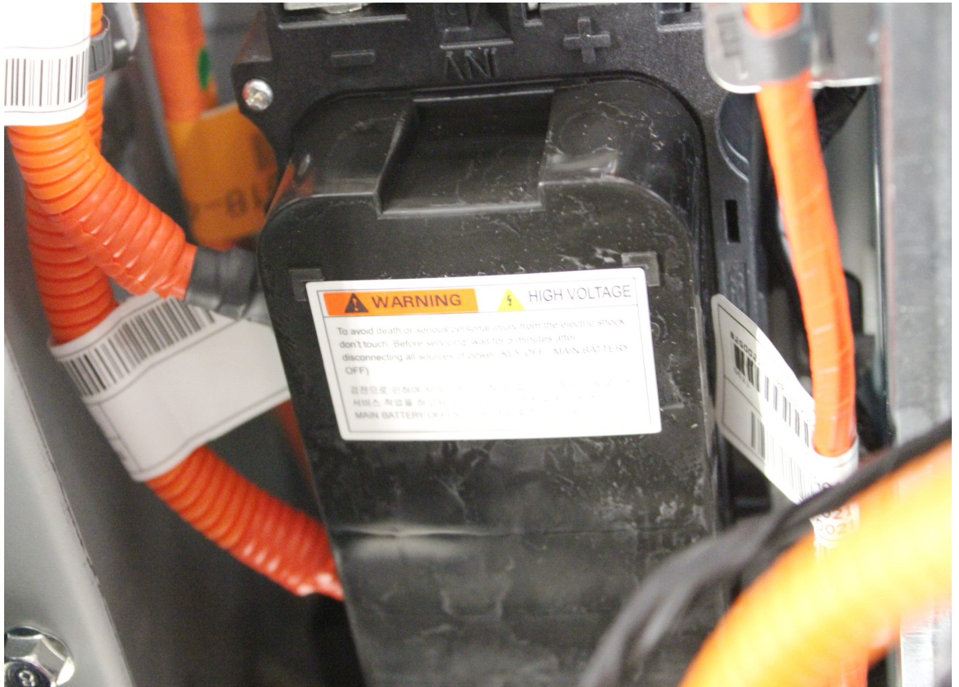
High Voltage Warning Label
