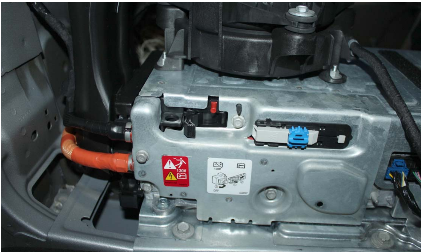
No. 007 Manual High Voltage Service Disconnect Removed
