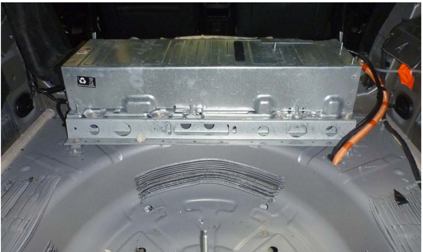
No. 011 Post-Impact Rear View Of Propulsion Battery
