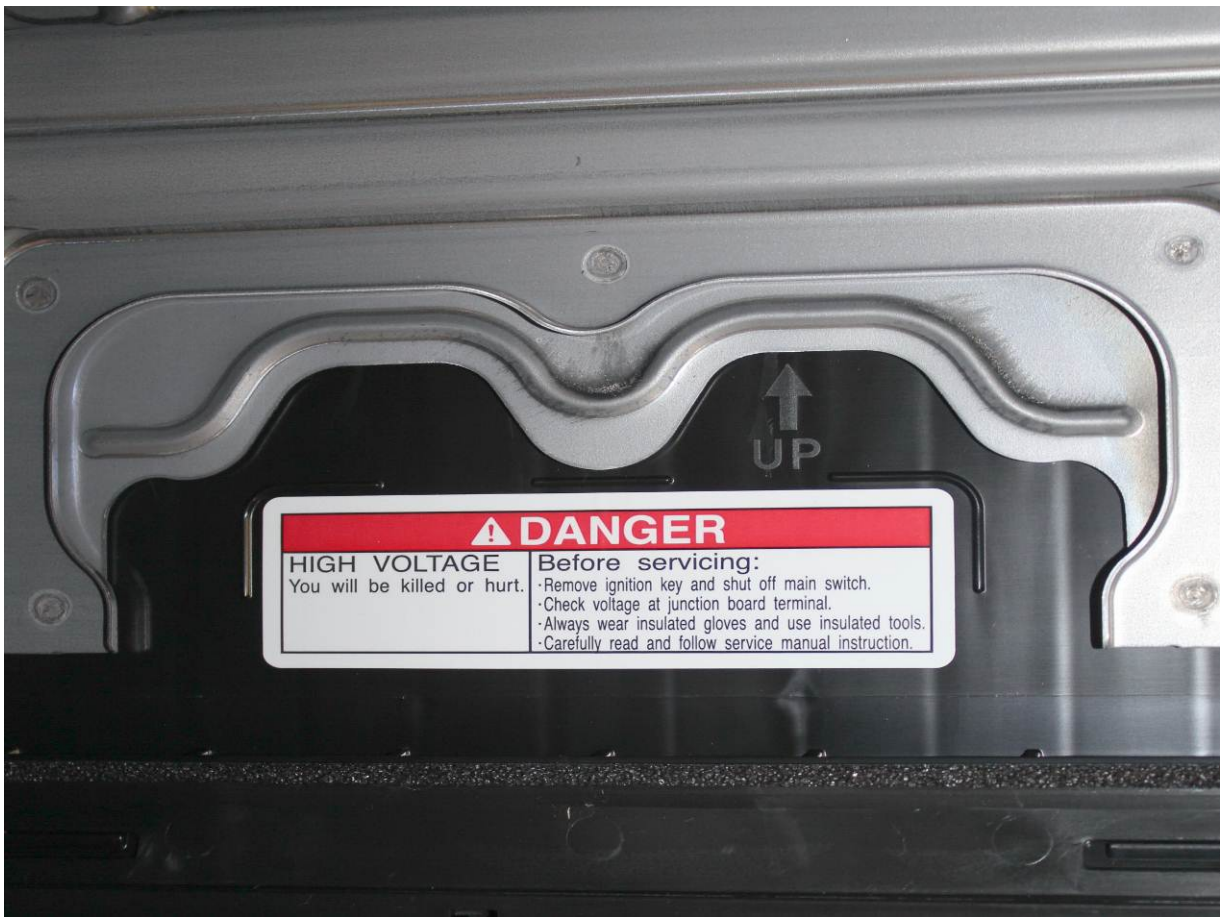
High Voltage Warning Label
