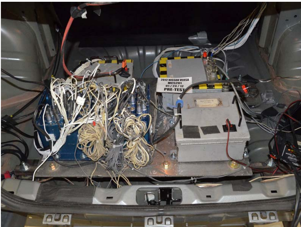
FIGURE 60. Pre-Test Ballast View
